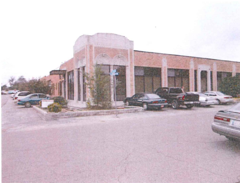
Photo 2- 8/24/12: South Eastern side of site.
