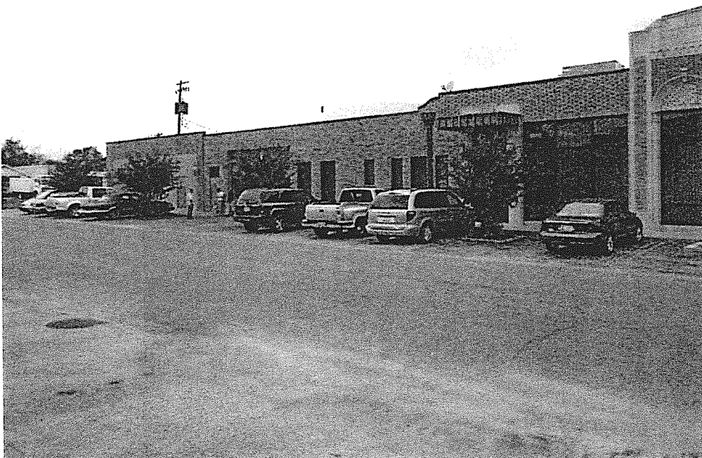
Photo 4- 8/24/12: South side of site.
