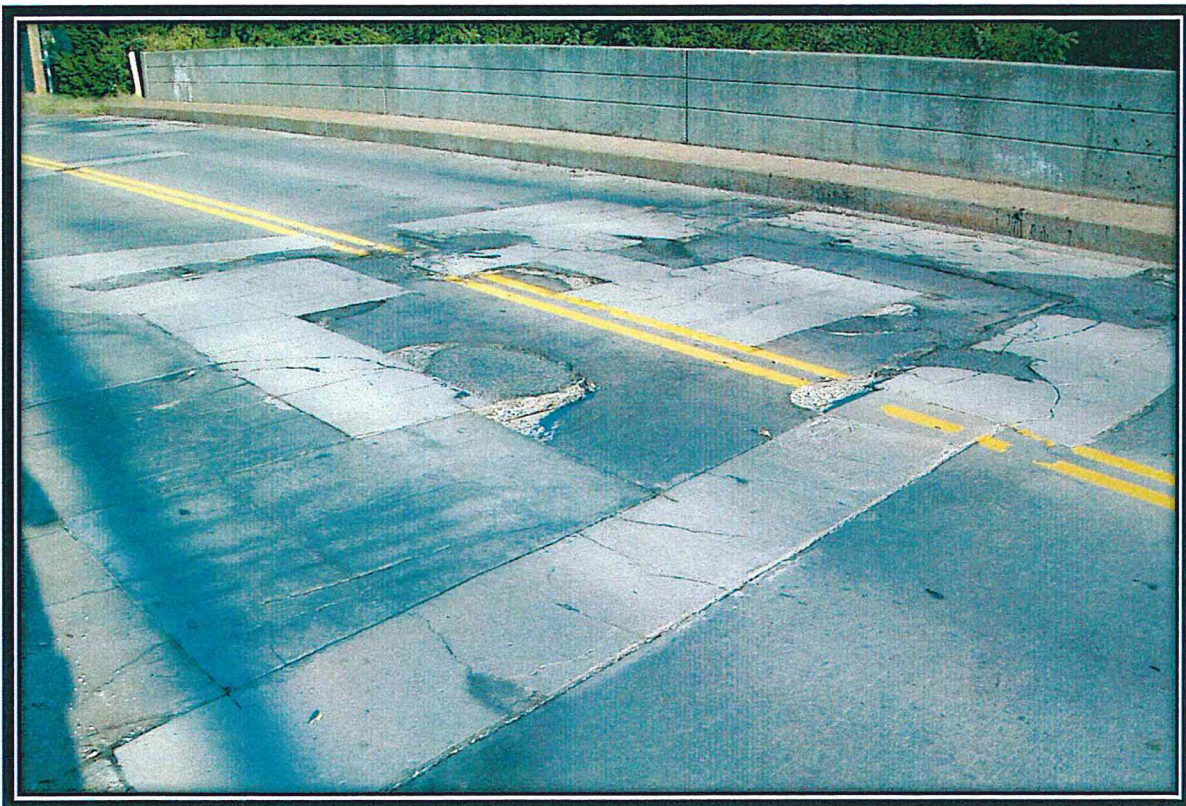
Condition of the Deck
