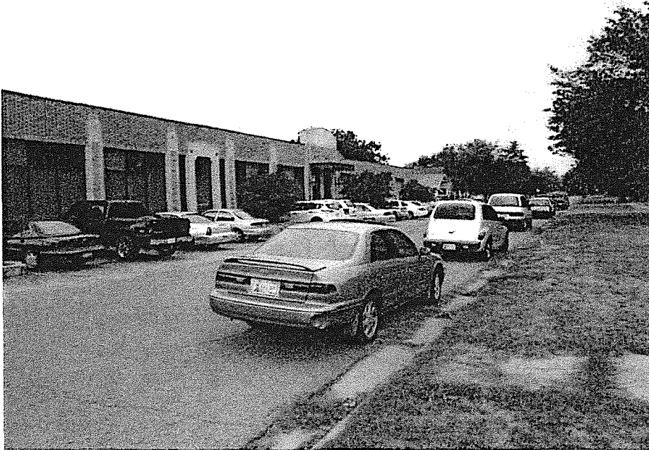
Photo 1 - 3/24/12: Eastern side of site.
