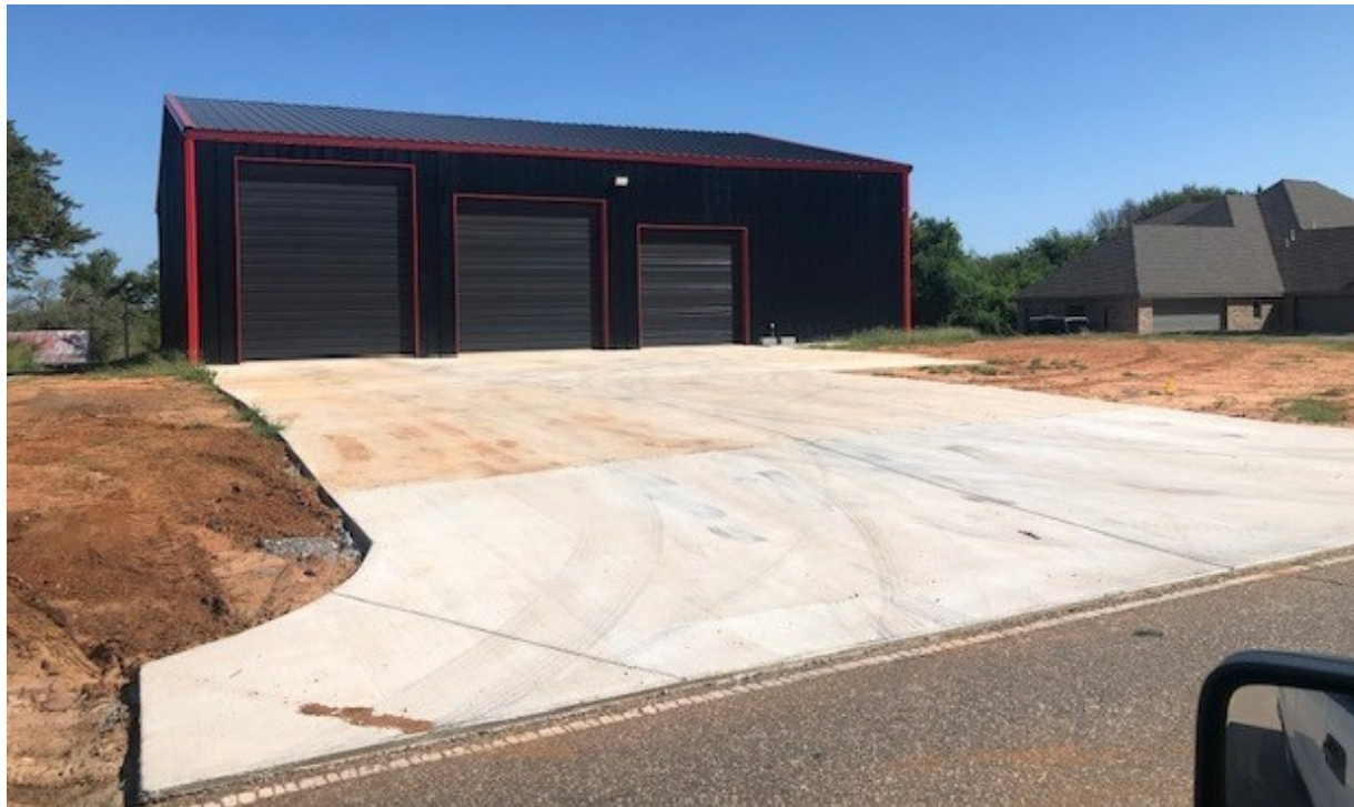
ZBOA04-21 -- 2130 W. Benedict St. (Top) existing west "house" driveway (Bottom) "new" accessory bldg. driveway
