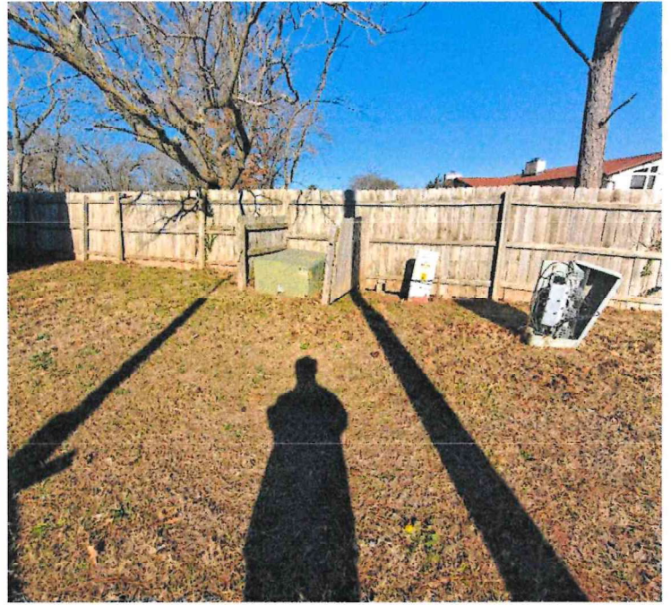
North Side Infrastructure Dec 2025
