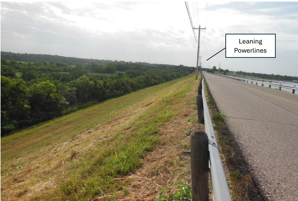
Photo No. 15: Looking east across the crest and downstream slope. Notice a slight angle to the powerlines.
