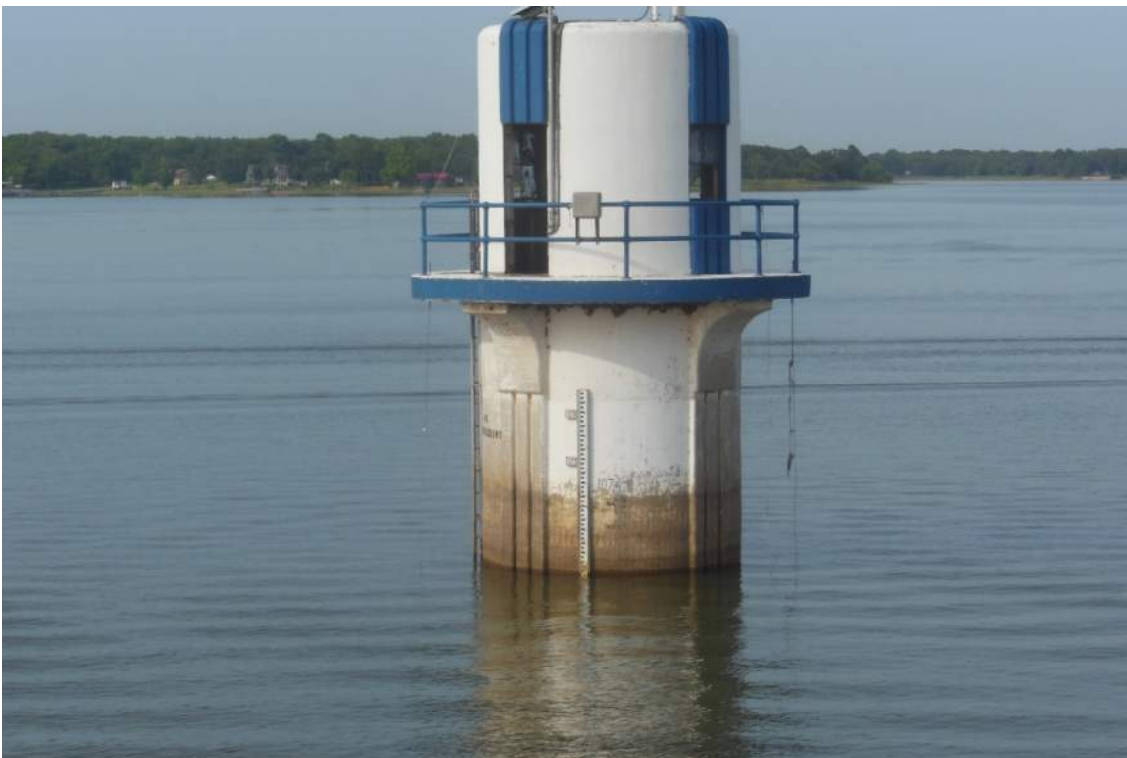
Photo No. 13: View of the intake tower from the upstream slope. During inspection, the water level was at approximate elevation 1072 ft, about 3ft lower than normal pool.
