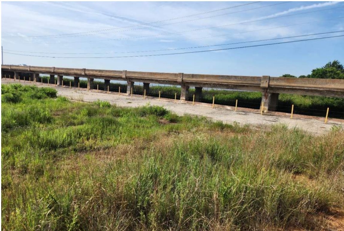
Photo No. 23: Looking upstream at the spillway crest.
