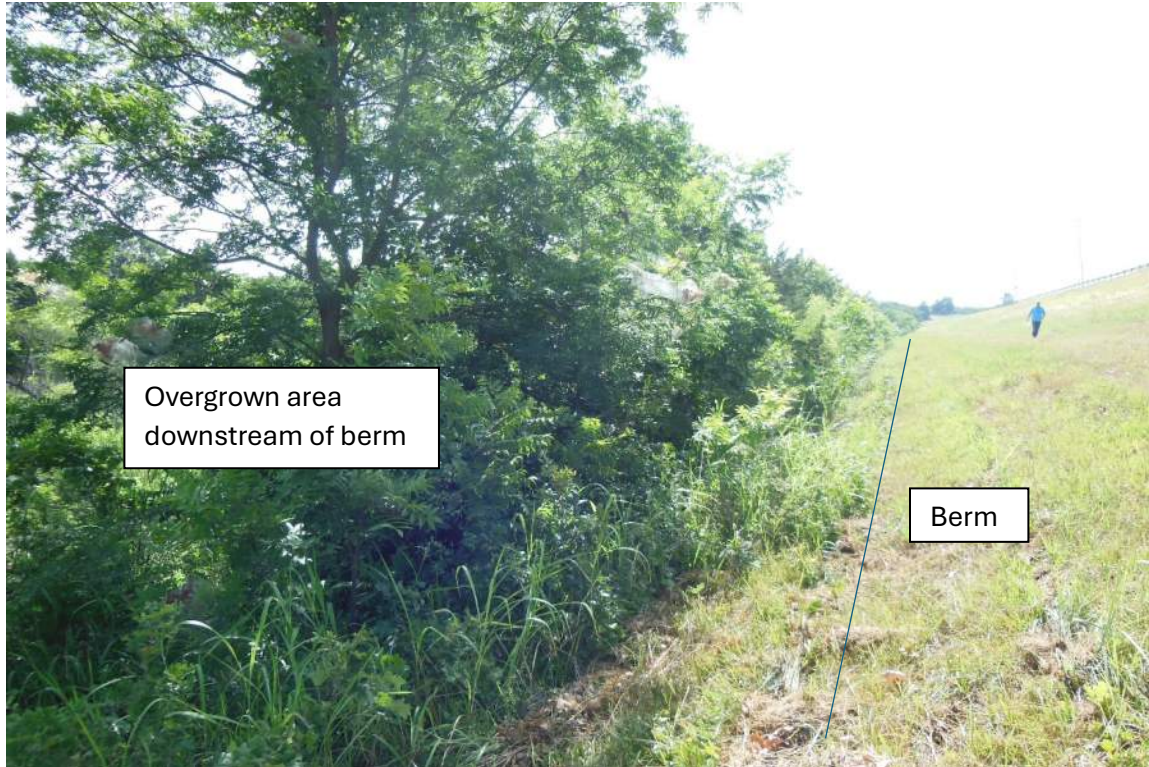
Photo No. 18: Looking east along the downstream berm. The area below the berm was not easily visible for inspection.
