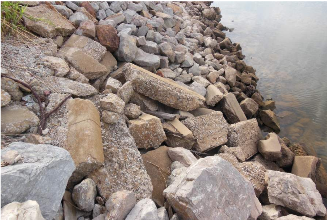
Photo No. 9: View of several large pieces of concrete among the riprap on the upstream slope.
