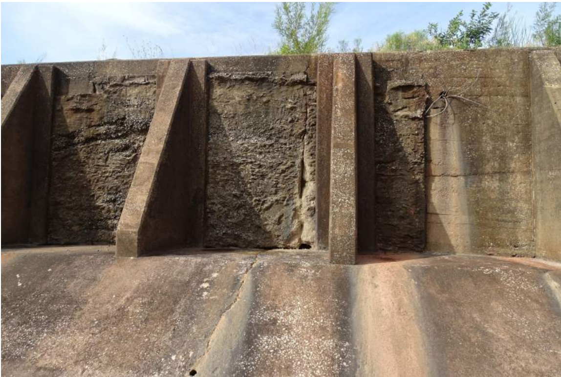
Photo No. 31: View of the downstream side of the stilling basin back wall and buttresses.
