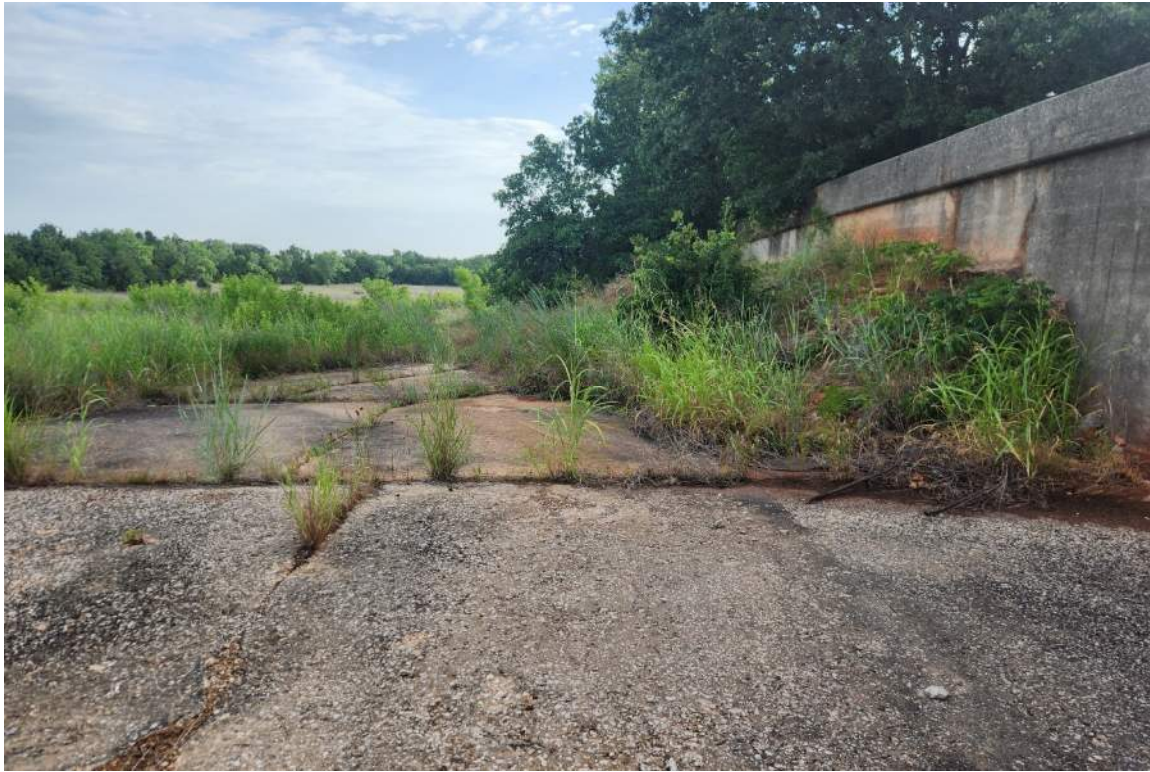
Photo No. 24: View of right spillway training wall looking downstream.
