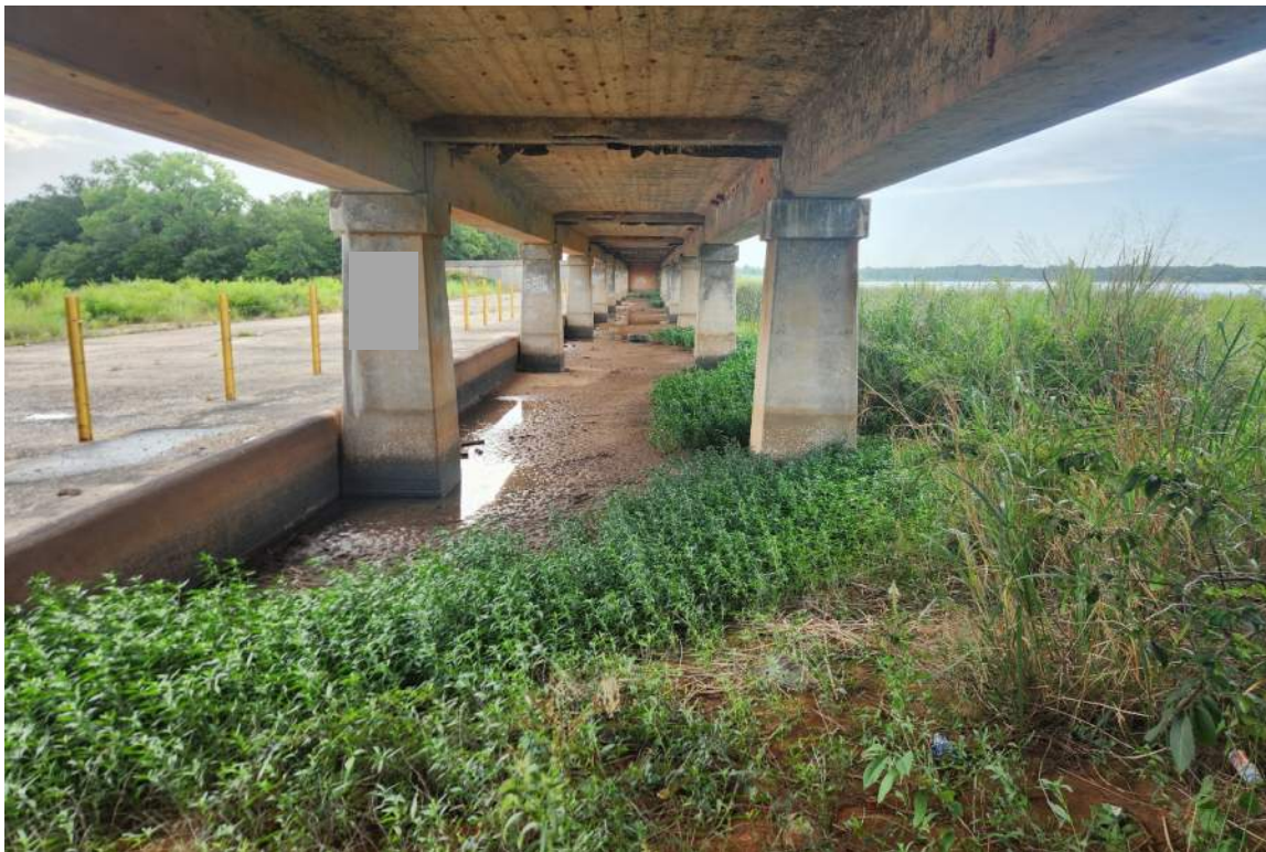
Photo No. 21: View of the spillway area under the bridge.
