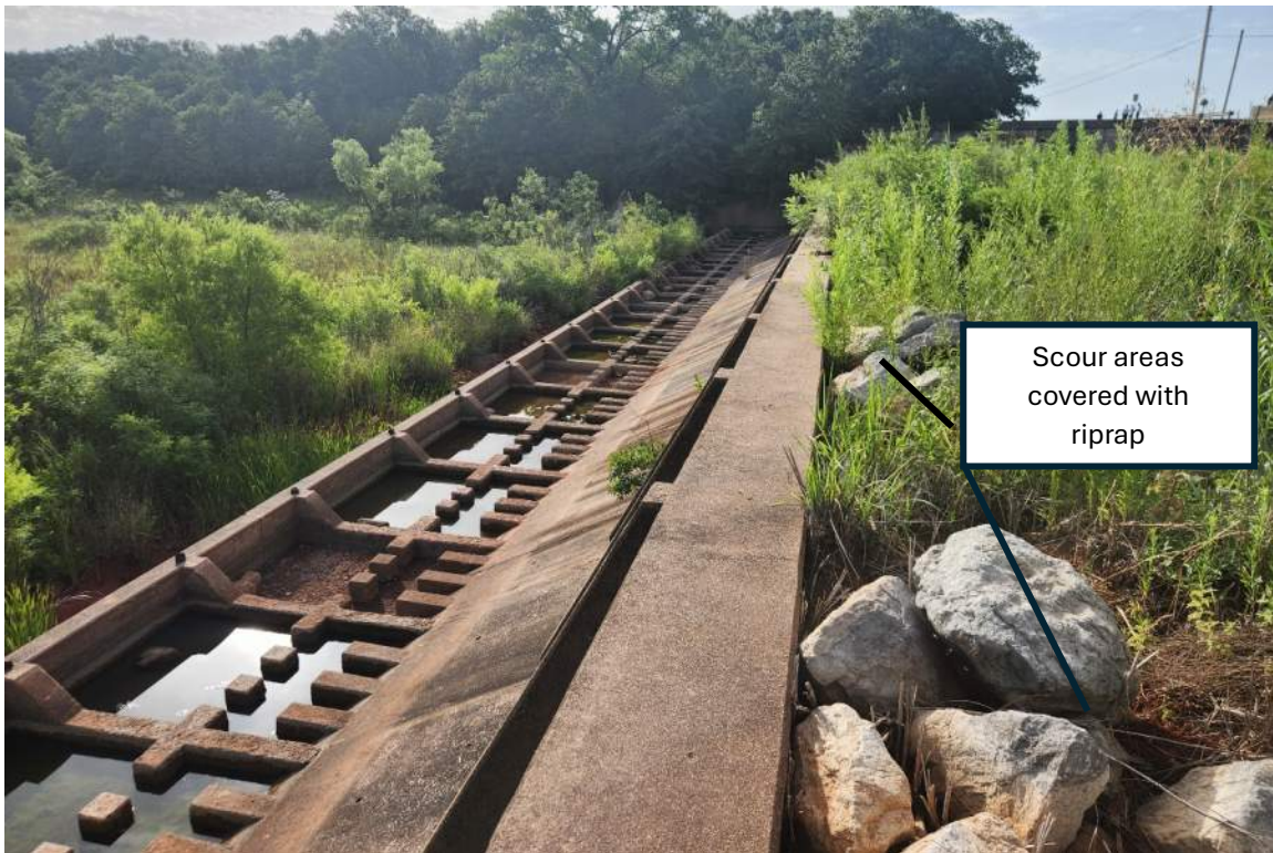
Photo No. 25: View of the flip bucket spilling basin. Notice the localized scour just upstream of the structure that has been filled with riprap.
