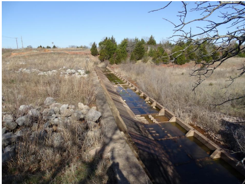
Figure 13. Riprap Scour Protection above the Flip Bucket Drop Structure
