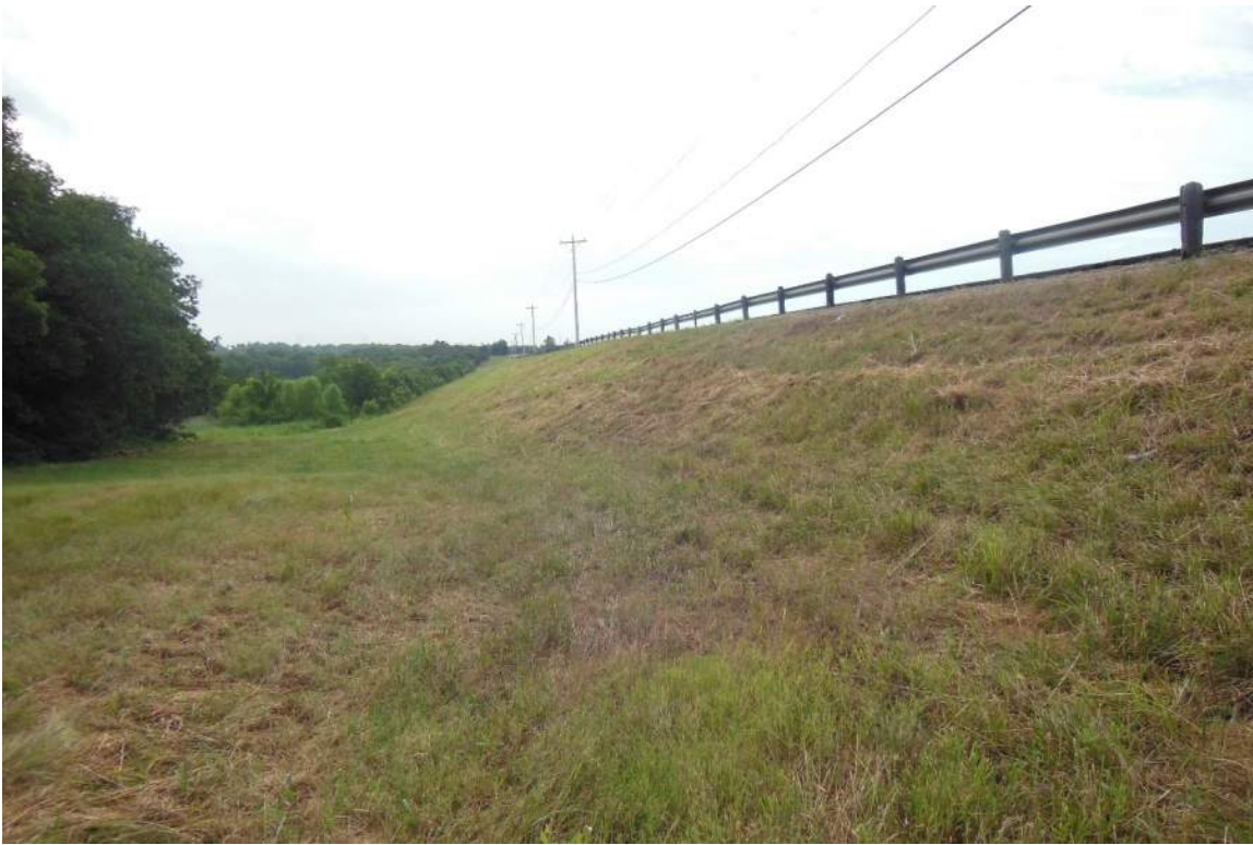
Photo No. 14: Looking east along the downstream slope from near the spillway.
