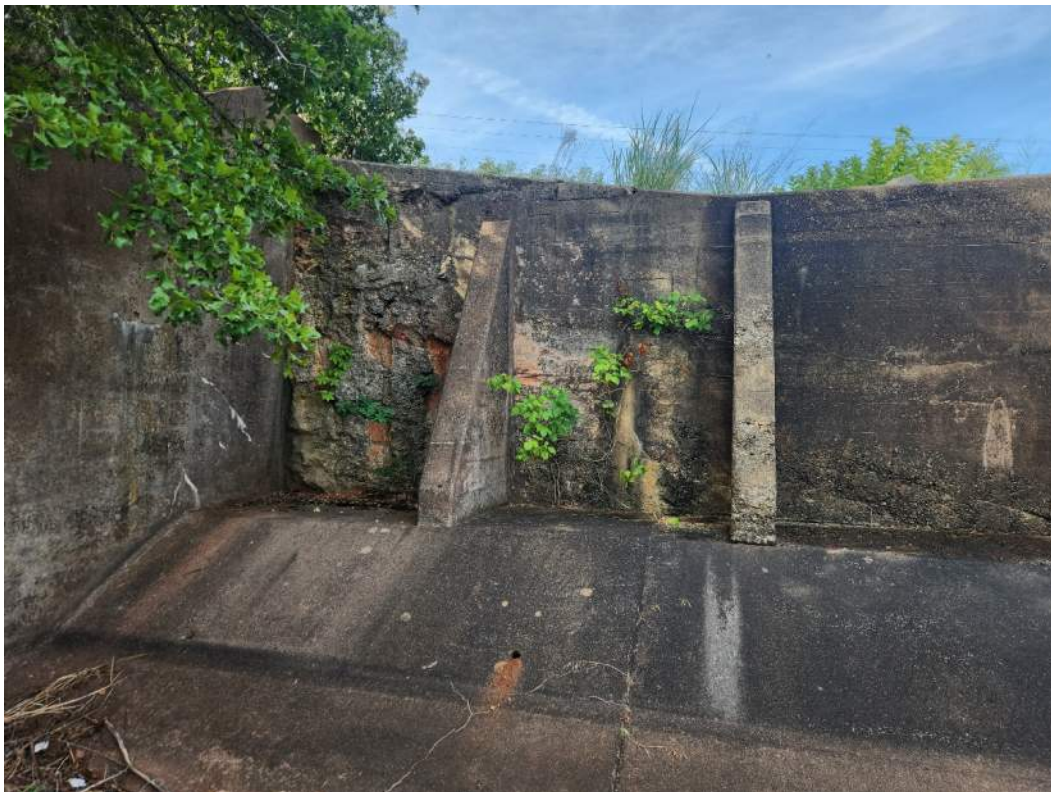
Photo No. 33: View of downstream side of right abutment of stilling basin structure.
