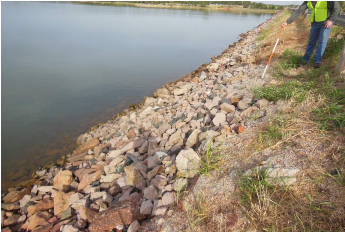
Photo No. 11: Looking west along the upstream slope.
