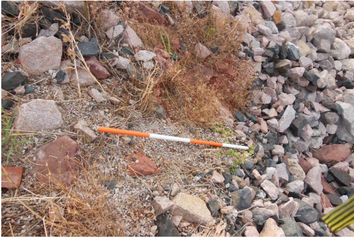
Photo No. 10: Finer grained aggregate and soil along the upstream slope near the crest.
