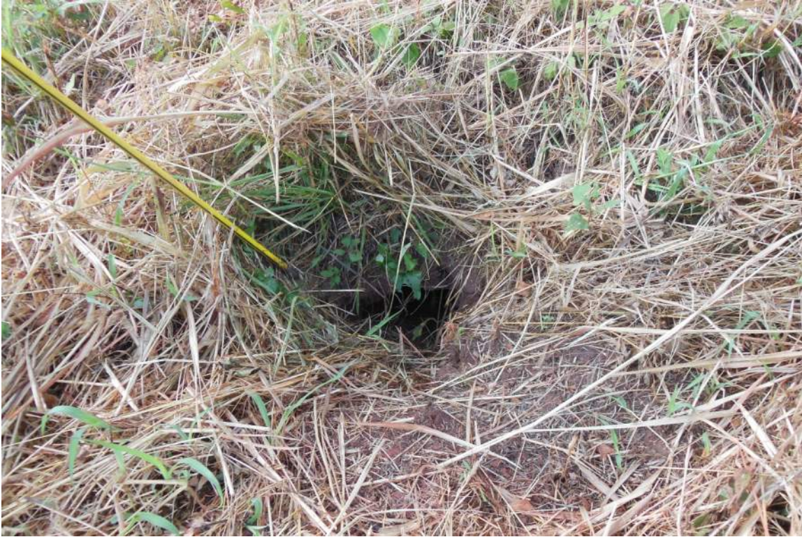
Photo No. 16: View of typical animal burrow along the downstream slope.
