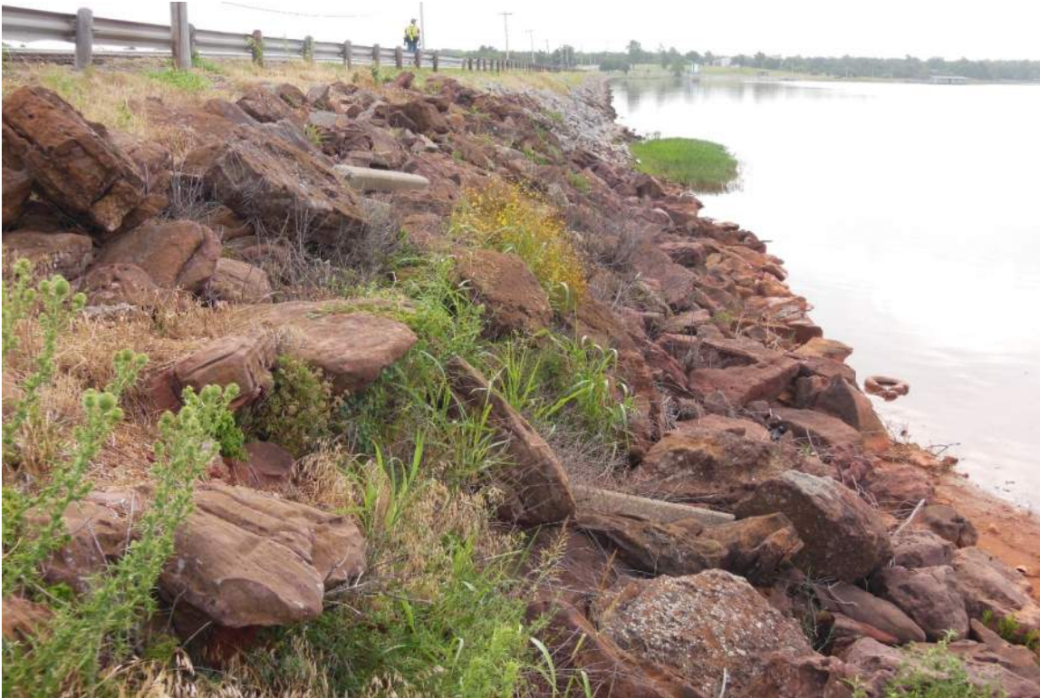
Photo No. 4: Looking east across the upstream slope from the left abutment.
