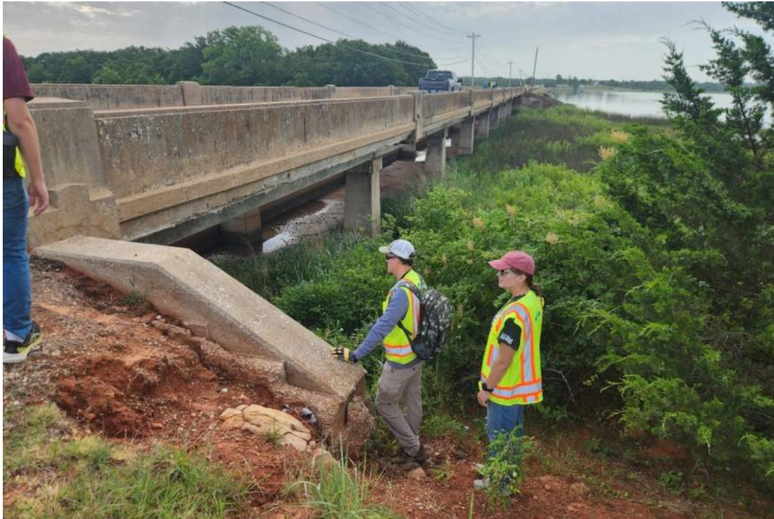
Photo No. 20: Looking east across the upstream side of the spillway.
