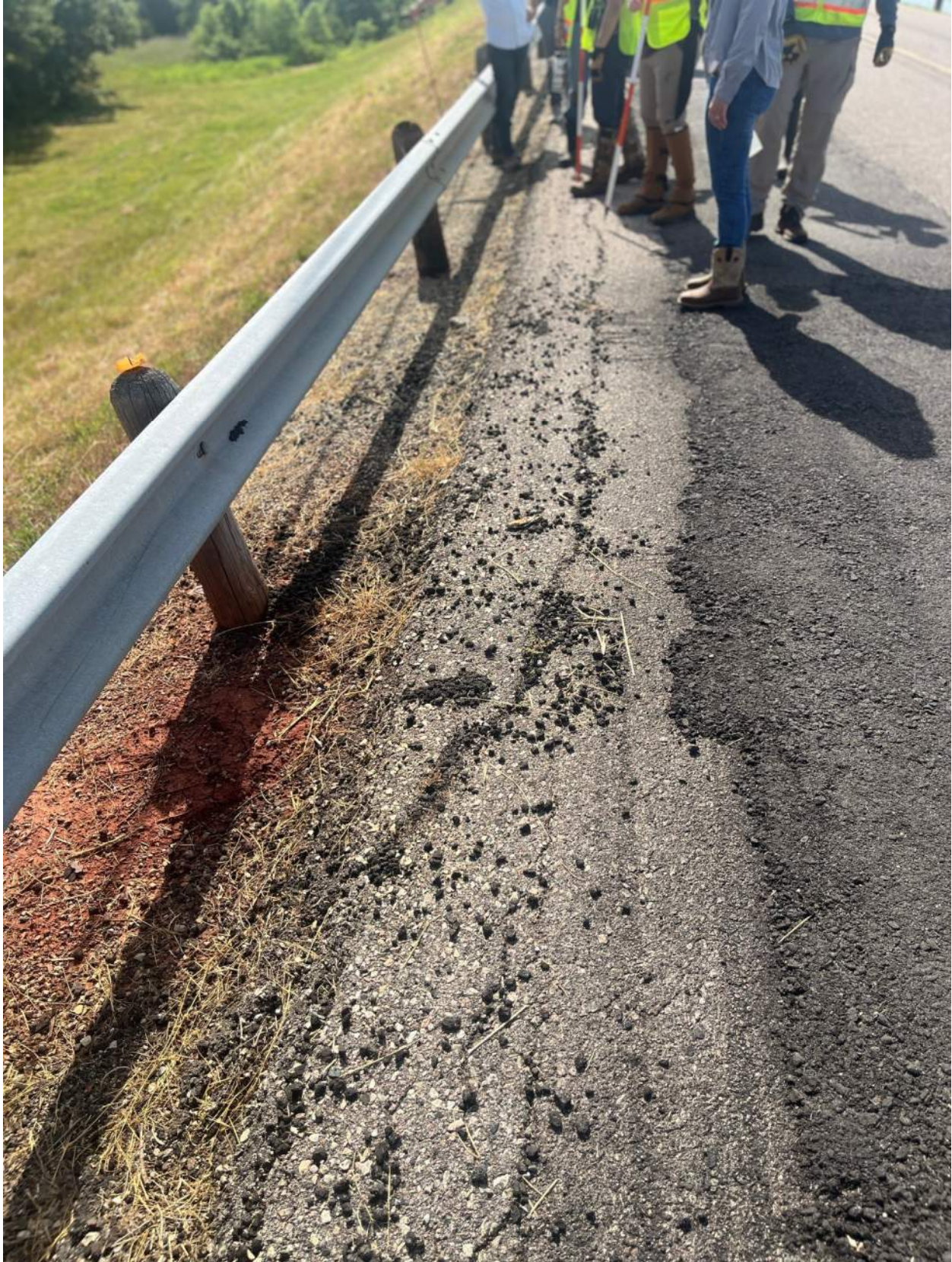
Photo No. 3: View of asphalt patch near spillway.
