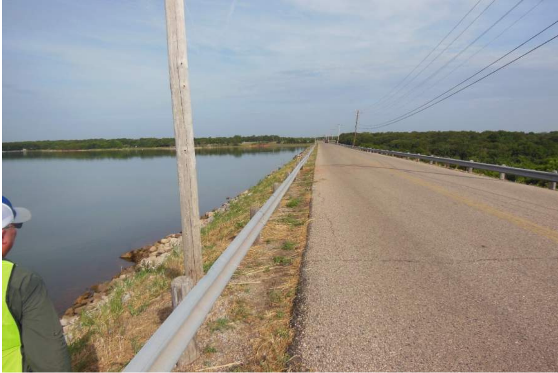
Photo No. 1: Looking west across the crest of dam
