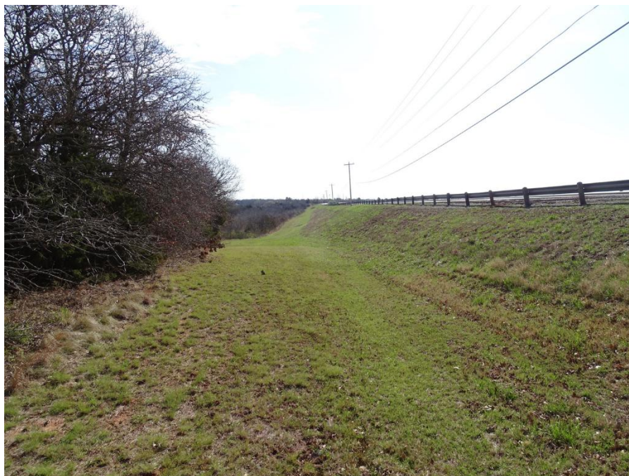
Figure 10. Downstream Slope in vicinity of the repaired roadway section (July 2024)
