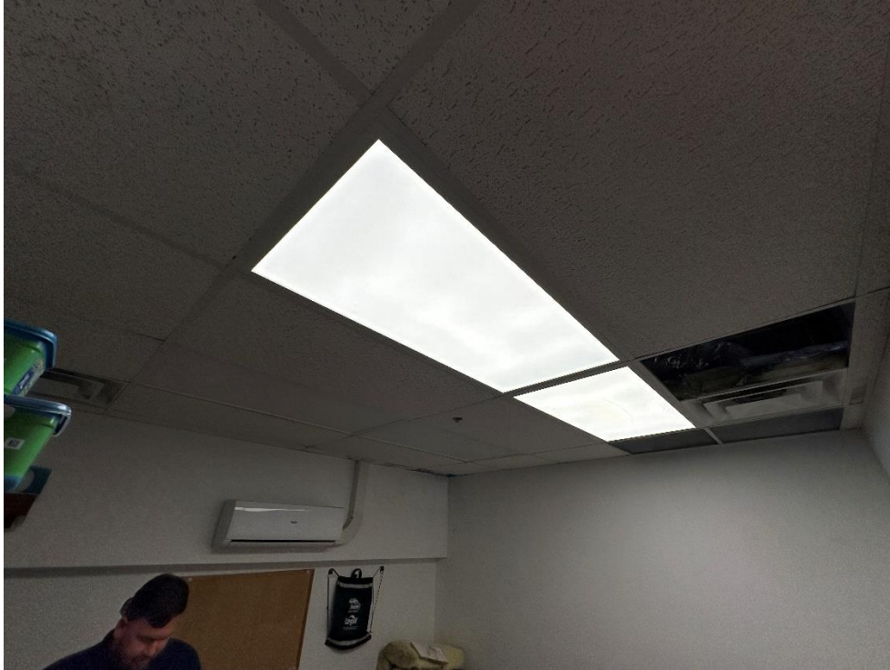
PHOTO #31: Overall view of the ceiling in the office.
