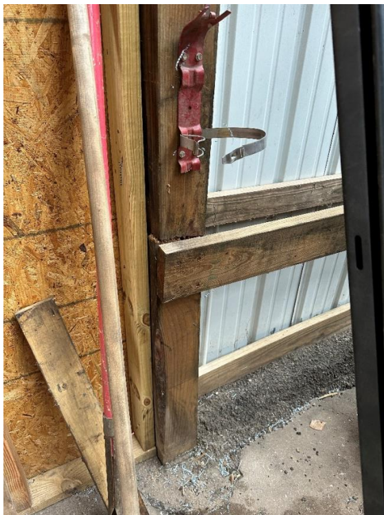
PHOTO #10: View of west end 6x6 broken wind column.
