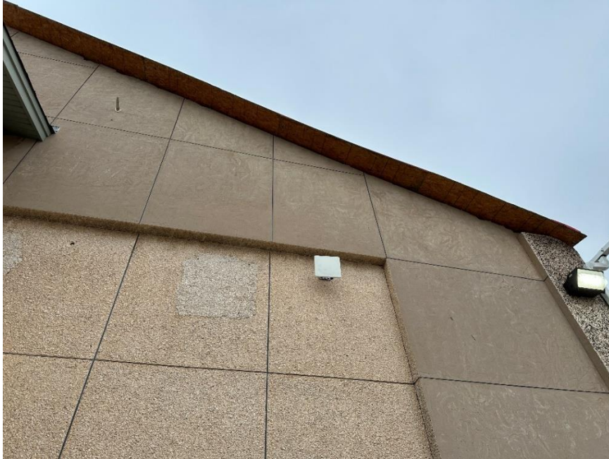
PHOTO #5: View looking north along south gable wall with removed soffit & outrigger materials under east gable end.
