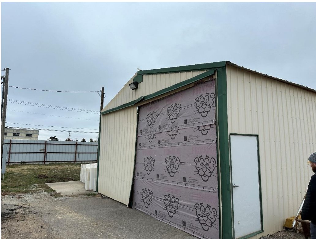
PHOTO #6: Sliding door removed, metal panels, trim and roof partially removed.
