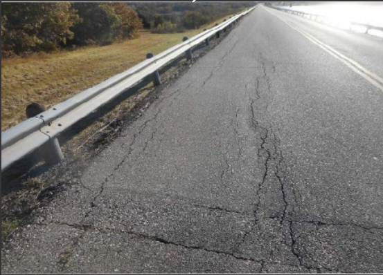
A slippage crack has developed in the upstream slope resulting in a depressed section about midway along the length of the dam.
