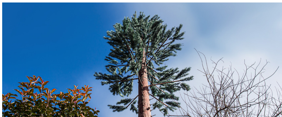
Telecommunication towers can be designed as trees to be camouflaged into the natural environment.
