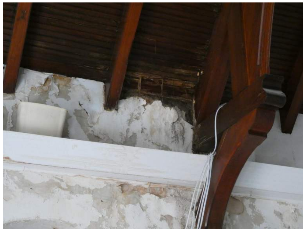
E EXISTING CONDITIONS PHOTO NOT TO SCALE
