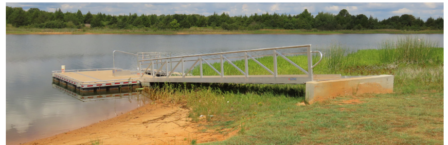
The kayak launch has an ADA accessible ramp and launch point. However, access to the launch is along a dirt path, and there is a 12-inch step to walk down the ramp.
