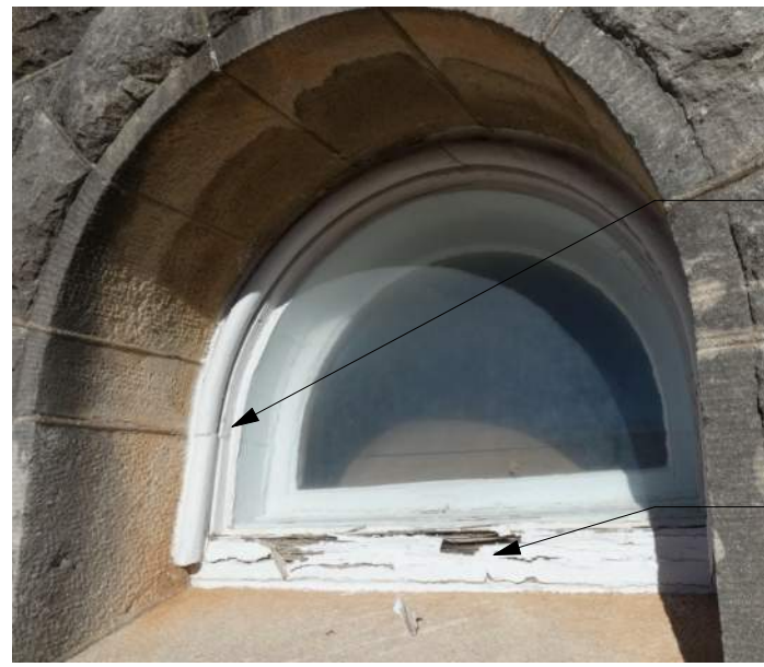
FIXED WOOD WINDOW (EAST ELEVATION)
