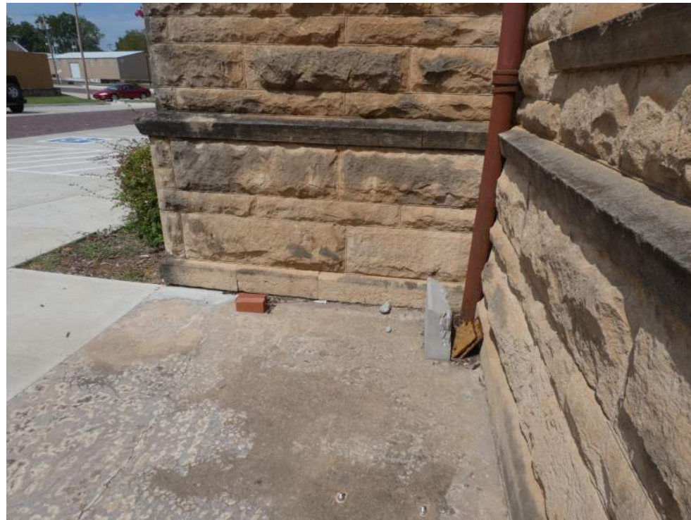
M EXISTING CONDITIONS PHOTO NOT TO SCALE
