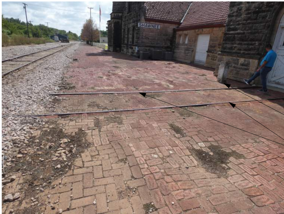
K EXISTING CONDITIONS PHOTO NOT TO SCALE
