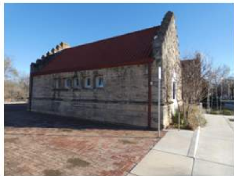
D EXISTING CONDITIONS PHOTO - NORTH NOT TO SCALE
