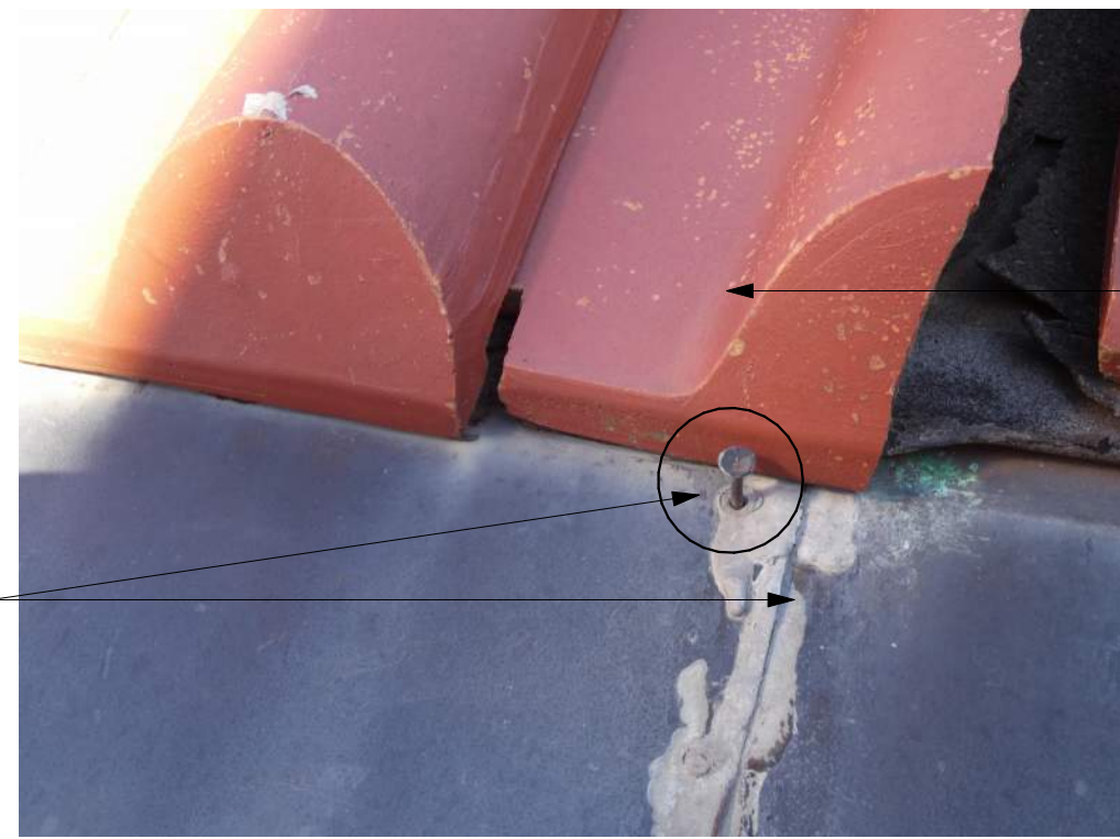
S EXISTING CONDITIONS PHOTO NOT TO SCALE
