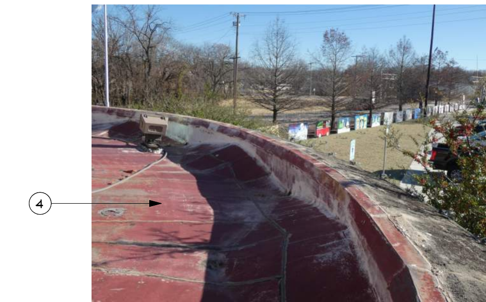
M EXISTING CONDITIONS PHOTOGRAPH NOT TO SCALE
