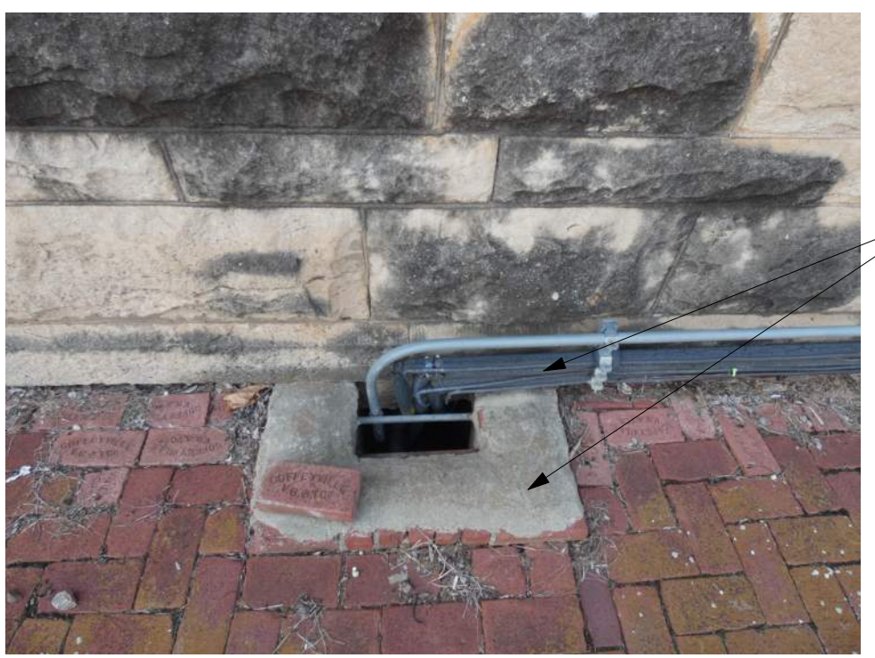
F EXISTING CONDITIONS PHOTO NOT TO SCALE
