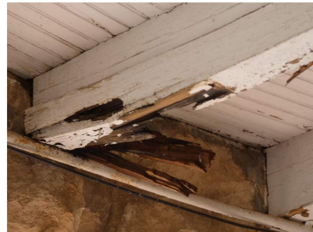
D EXISTING CONDITIONS PHOTO NOT TO SCALE
