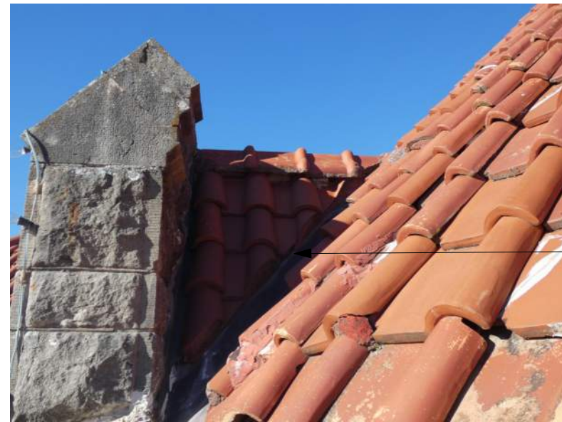
H EXISTING CONDITIONS PHOTOGRAPH NOT TO SCALE
