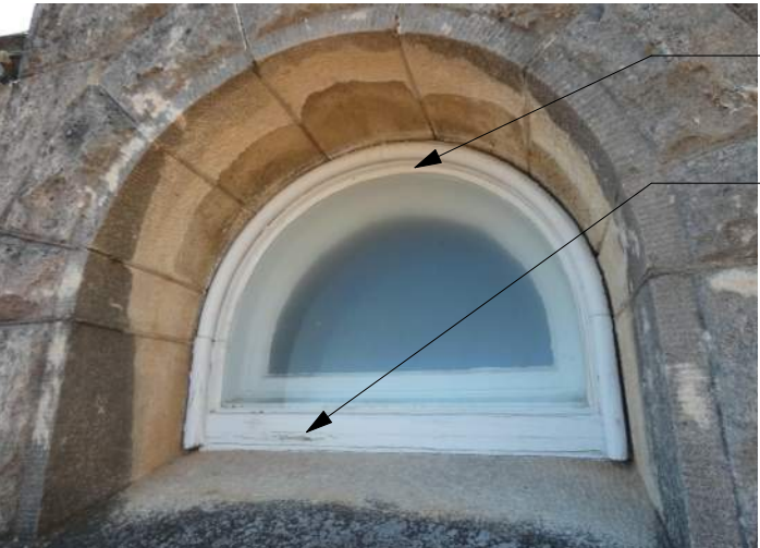
FIXED WOOD WINDOW (EAST ELEVATION)
