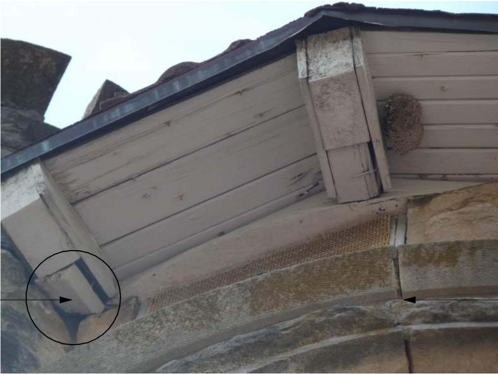
F EXISTING CONDITIONS PHOTO NOT TO SCALE
