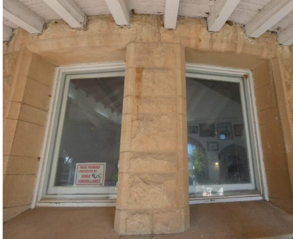
WOOD CASEMENT AT ROTUNDA
