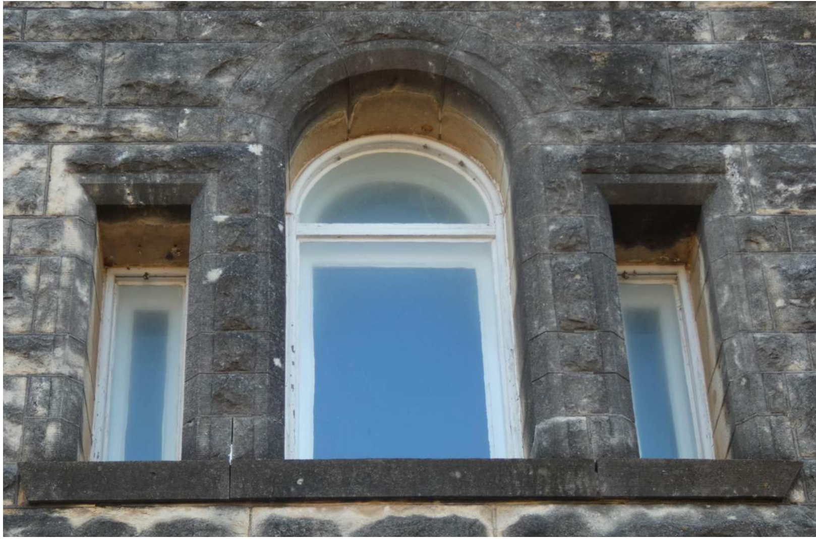
CASEMENT WOOD HOPPER AND CASEMENT CASEMENT
