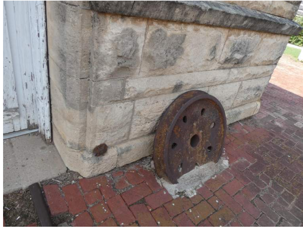
H EXISTING CONDITIONS PHOTO NOT TO SCALE
