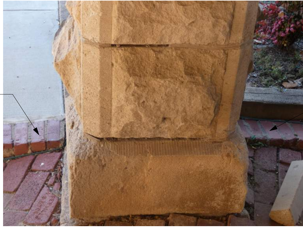
D EXISTING CONDITIONS PHOTO NOT TO SCALE
