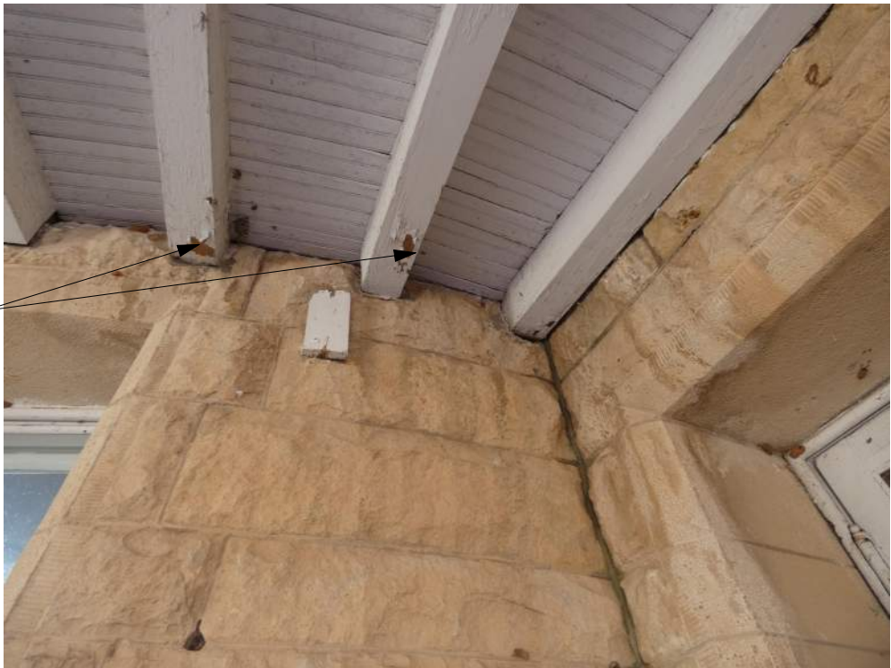
K EXISTING CONDITIONS PHOTO NOT TO SCALE
