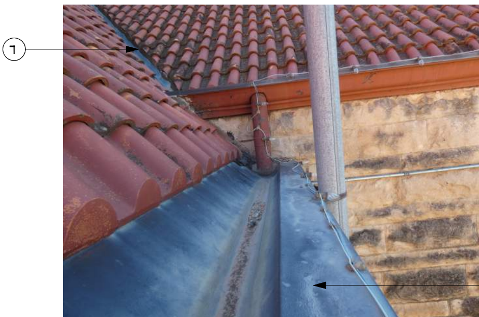
L EXISTING CONDITIONS PHOTOGRAPH NOT TO SCALE
