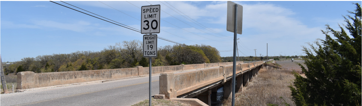
Larger roadway projects, such as bridge replacements, may not be included in the budget annually. A formalized Capital Improvements Plan (CIP) process can help a city plan out budgetary needs for the subsequent five to ten years.
