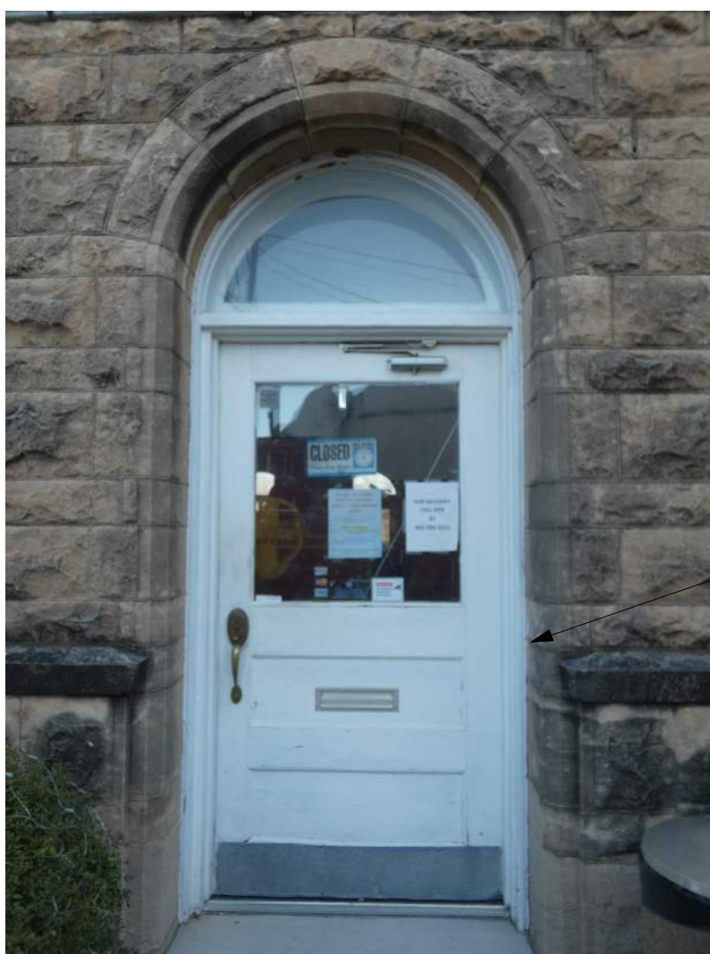
WEST DOOR AND WOOD TRANSOM
