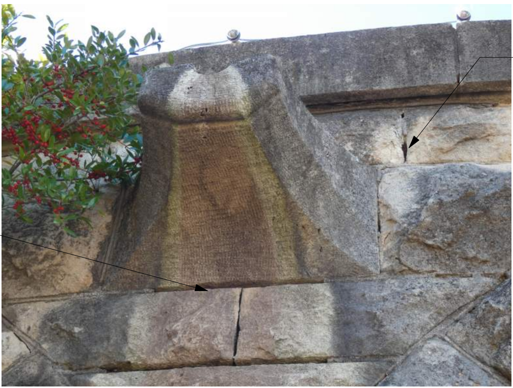
M EXISTING CONDITIONS PHOTO NOT TO SCALE
