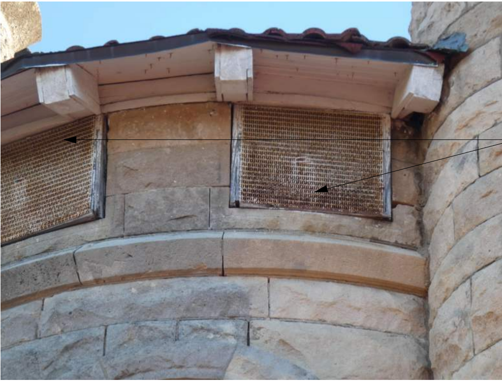
E EXISTING CONDITIONS PHOTO NOT TO SCALE
