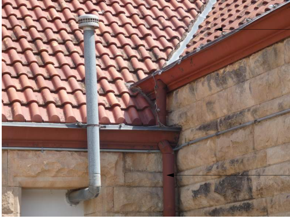
R EXISTING CONDITIONS PHOTO NOT TO SCALE
