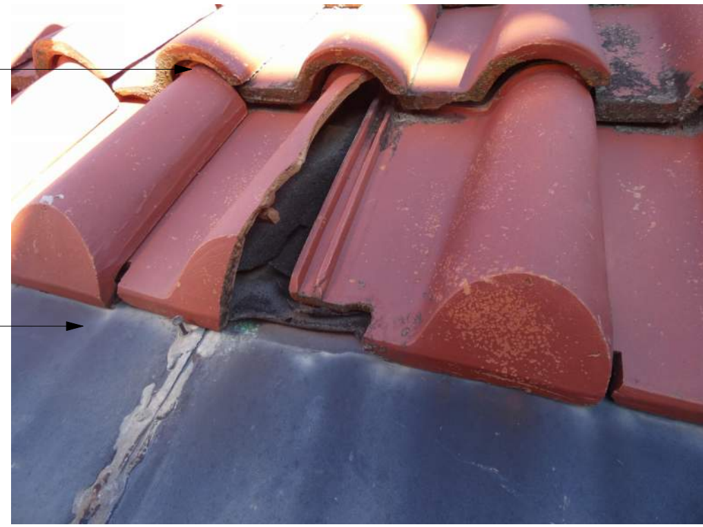
M EXISTING CONDITIONS PHOTO NOT TO SCALE
