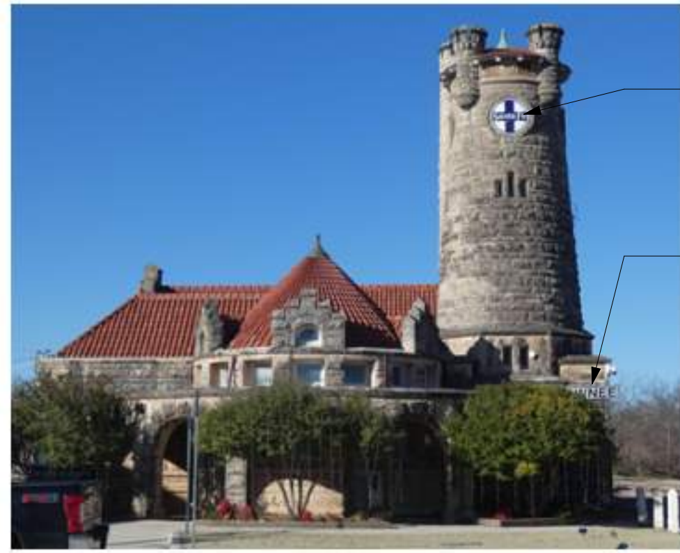
F EXISTING CONDITIONS PHOTO - SOUTH NOT TO SCALE
