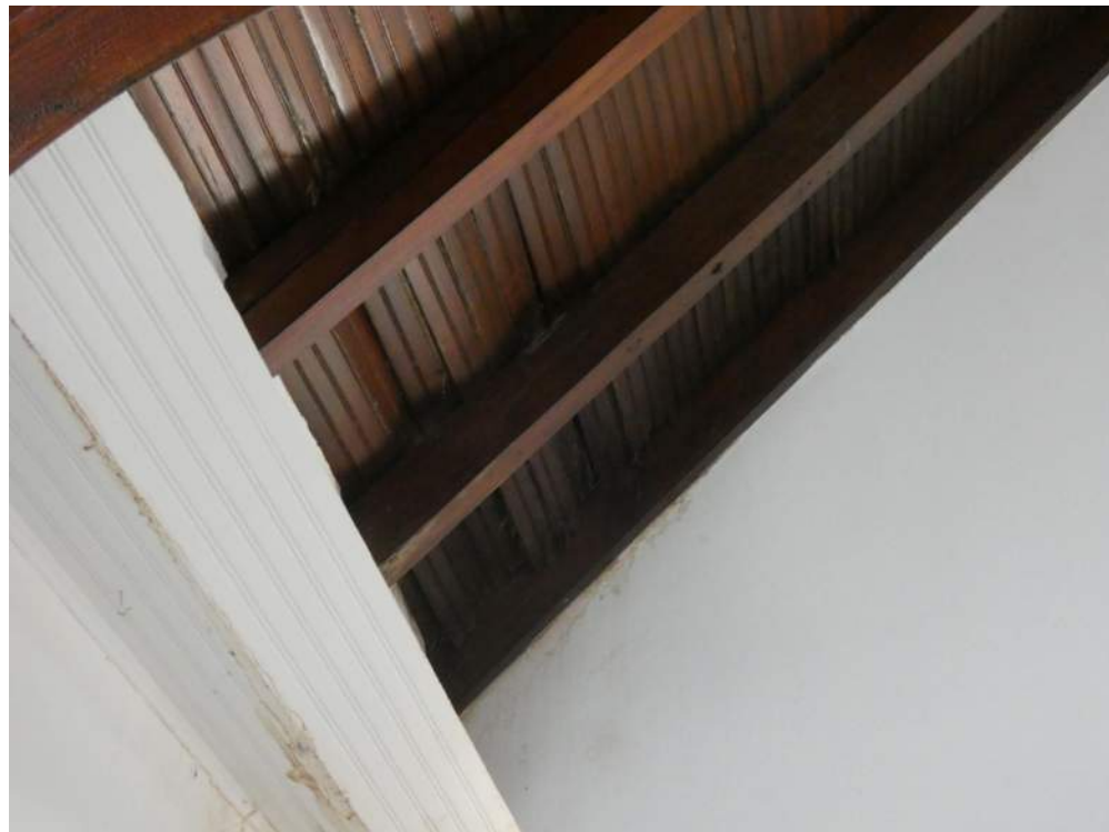
F EXISTING CONDITIONS PHOTO NOT TO SCALE
