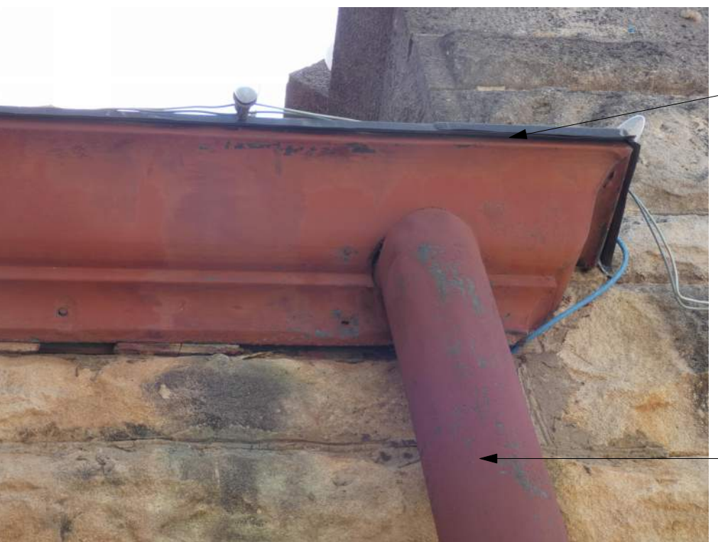
F EXISTING CONDITIONS PHOTO NOT TO SCALE
