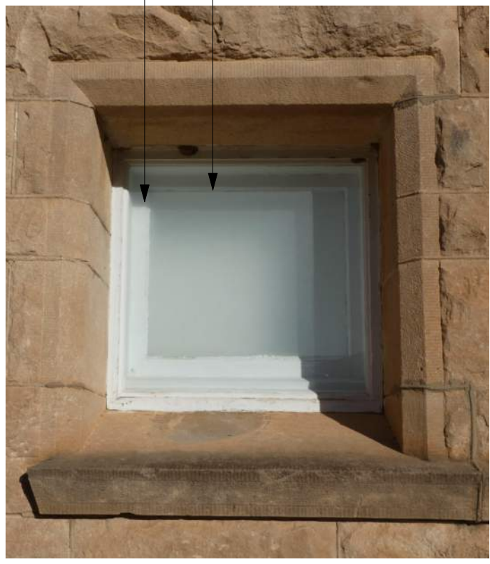
BOARDED UP WINDOW (WEST SIDE)
