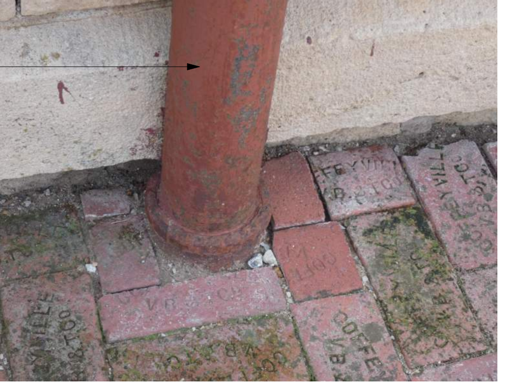
E EXISTING CONDITIONS PHOTO NOT TO SCALE
