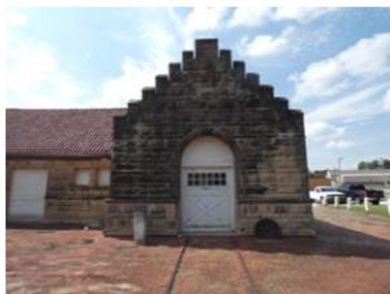
F EXISTING CONDITIONS PHOTO - EAST NOT TO SCALE
