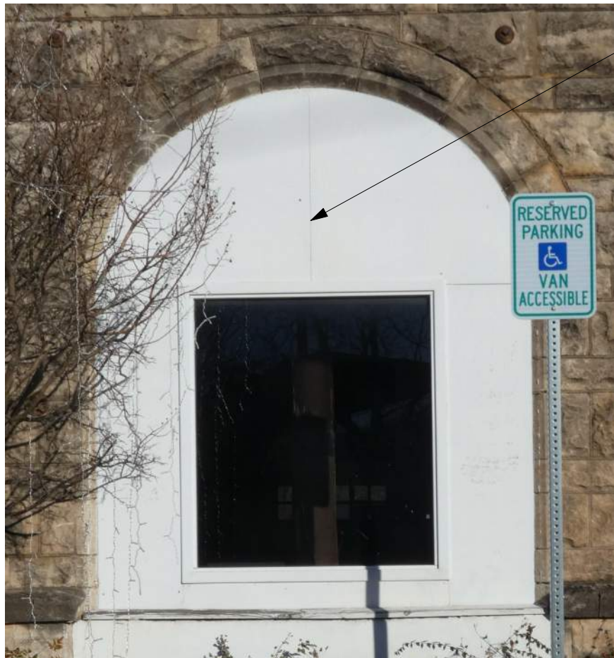
FIXED INFILL FOR WEST SLIDING DOOR
