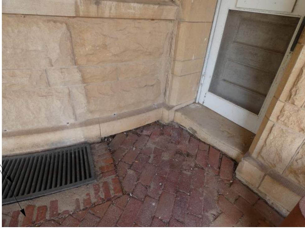
B EXISTING CONDITIONS PHOTO NOT TO SCALE
