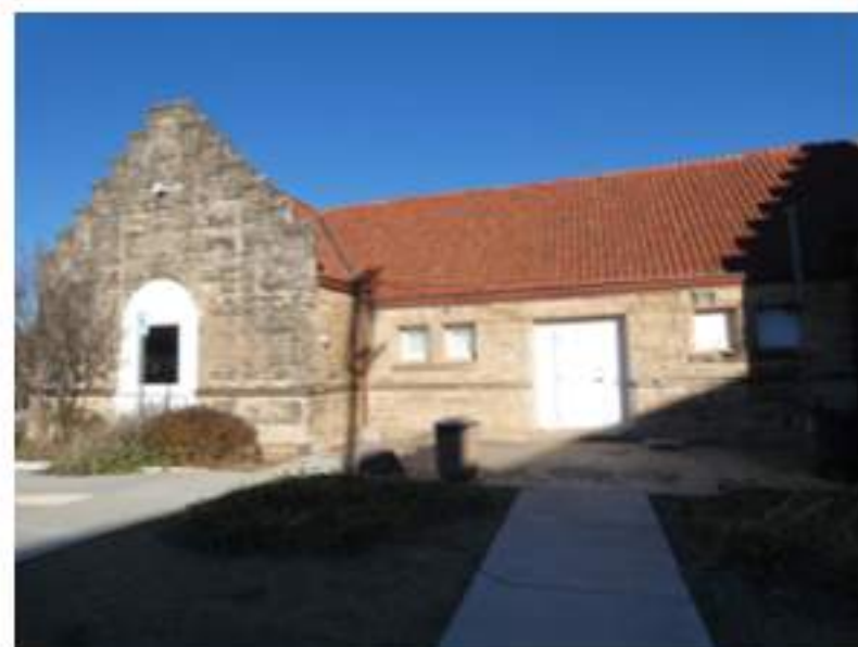
E EXISTING CONDITIONS PHOTO - WEST NOT TO SCALE
