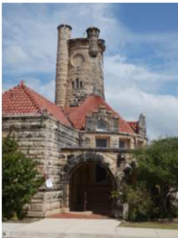
C EXISTING CONDITIONS PHOTO - WEST NOT TO SCALE
