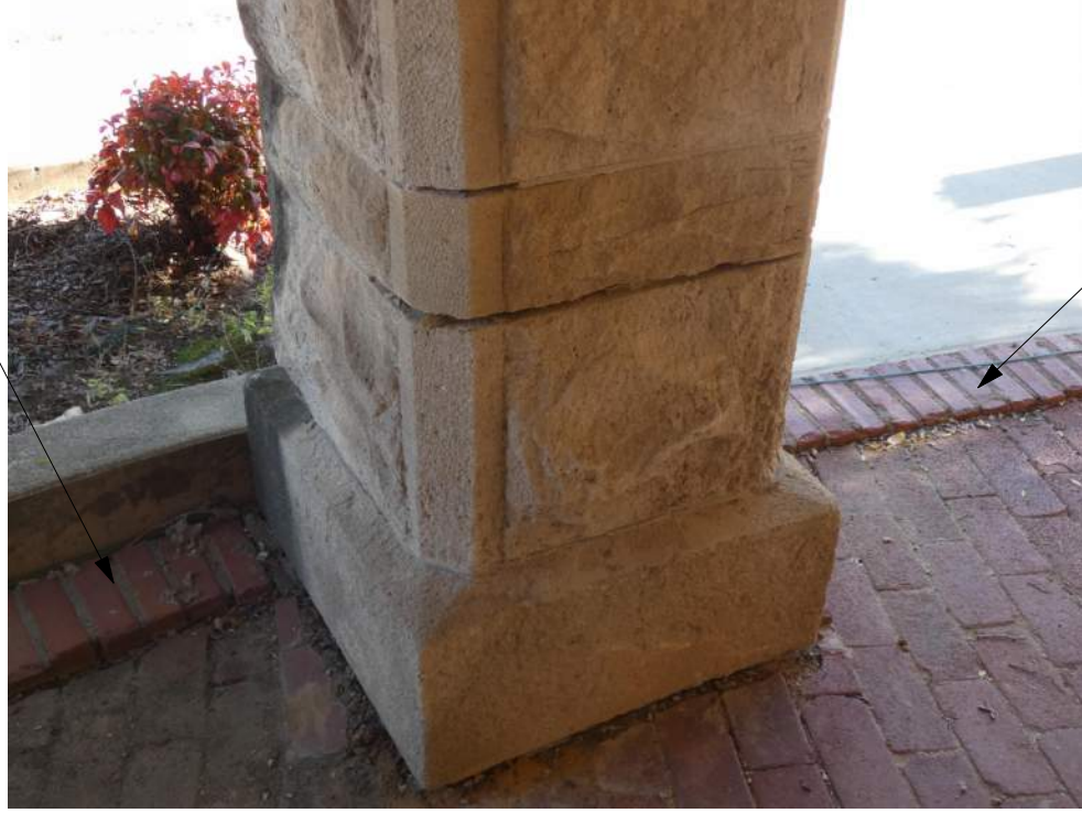
P EXISTING CONDITIONS PHOTO NOT TO SCALE
