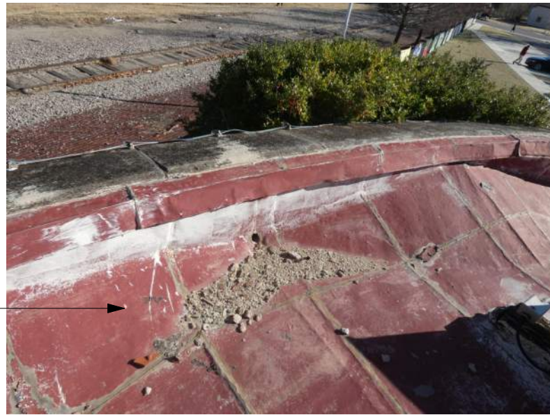
J EXISTING CONDITIONS PHOTOGRAPH NOT TO SCALE
