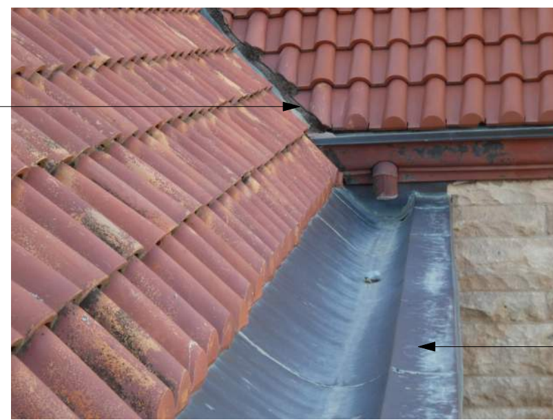
F EXISTING CONDITIONS PHOTOGRAPH NOT TO SCALE
