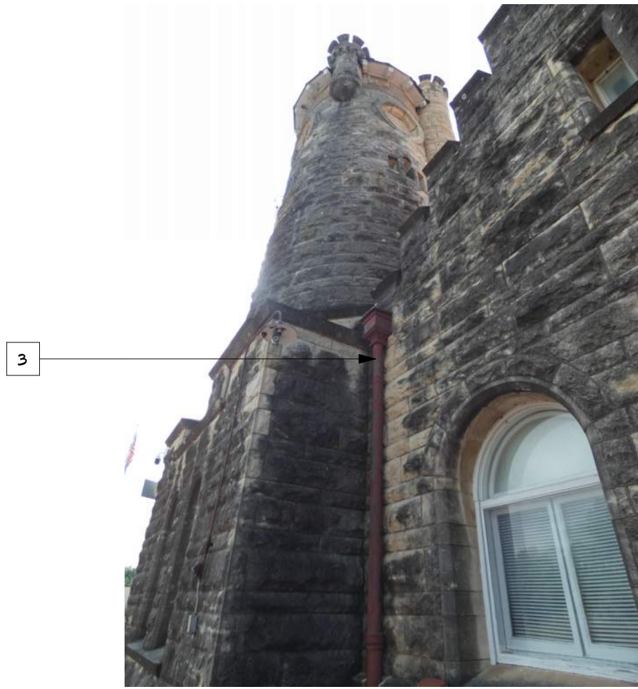
P EXISTING CONDITIONS PHOTO NOT TO SCALE
