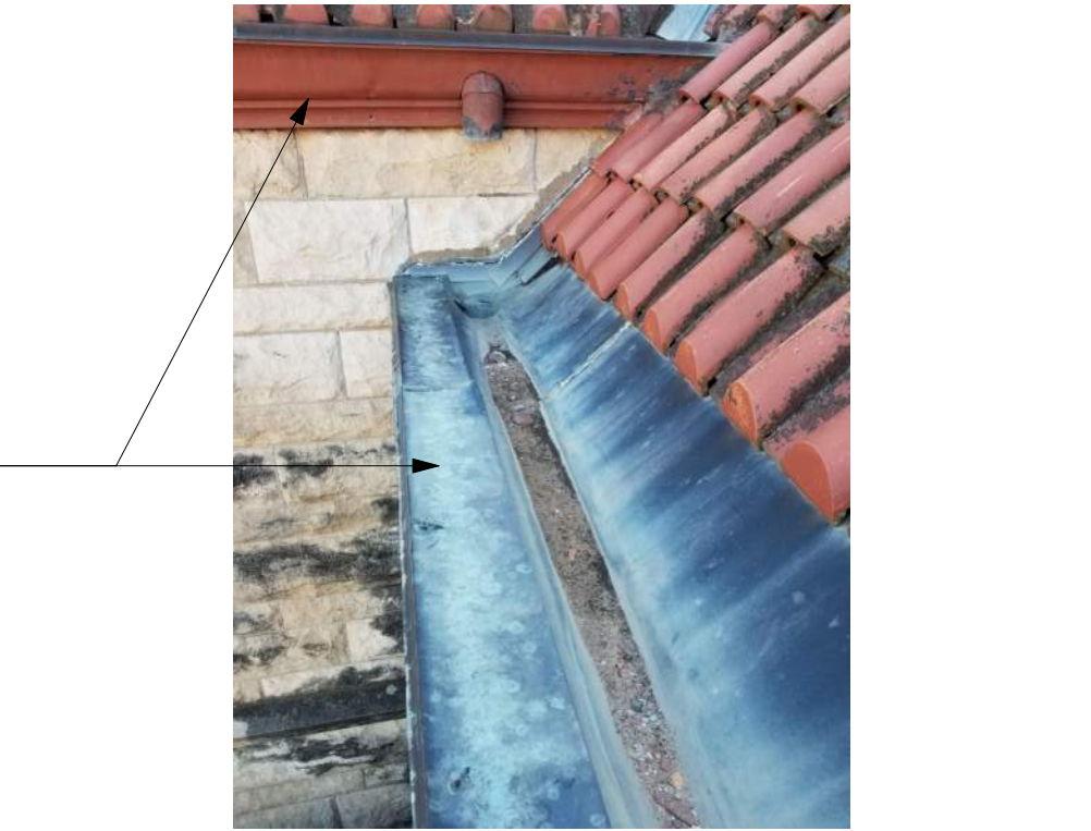
H EXISTING CONDITIONS PHOTO NOT TO SCALE
