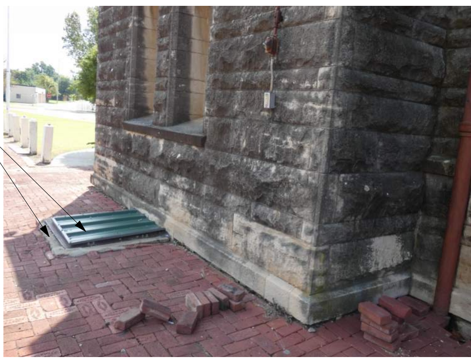
E EXISTING CONDITIONS PHOTO NOT TO SCALE
