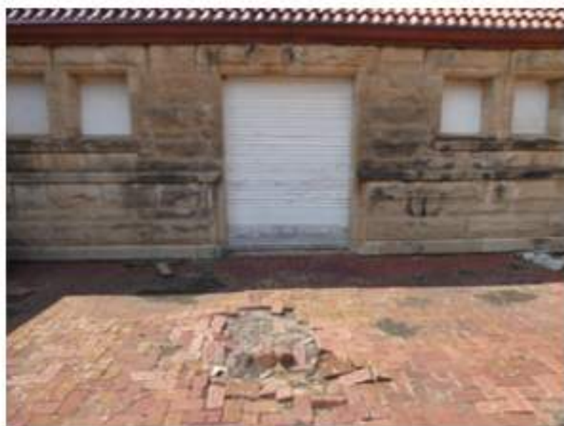
G EXISTING CONDITIONS PHOTO - EAST NOT TO SCALE
