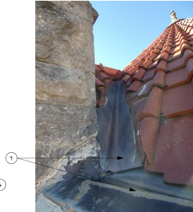
C EXISTING CONDITIONS PHOTOGRAPH NOT TO SCALE
