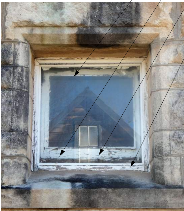
CASEMENT NORTH WINDOW
