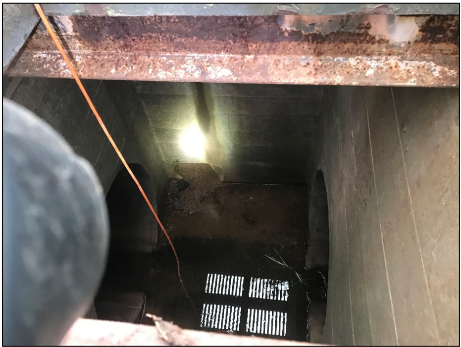
Figure 4: Inside of Grate Inlet
