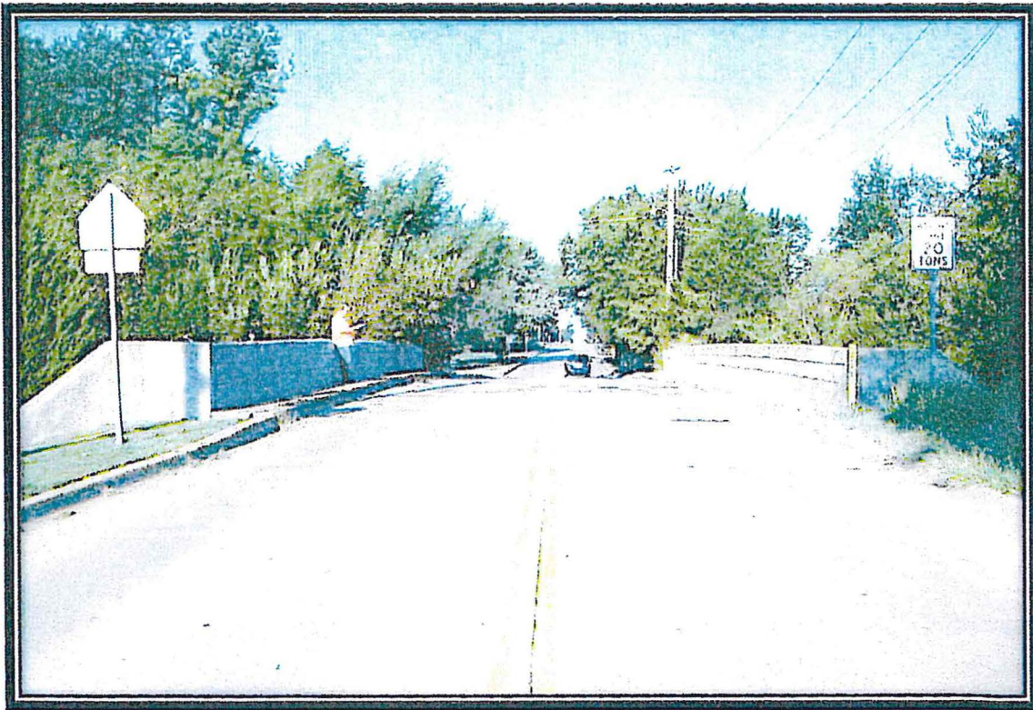
Looking West along the deck.
