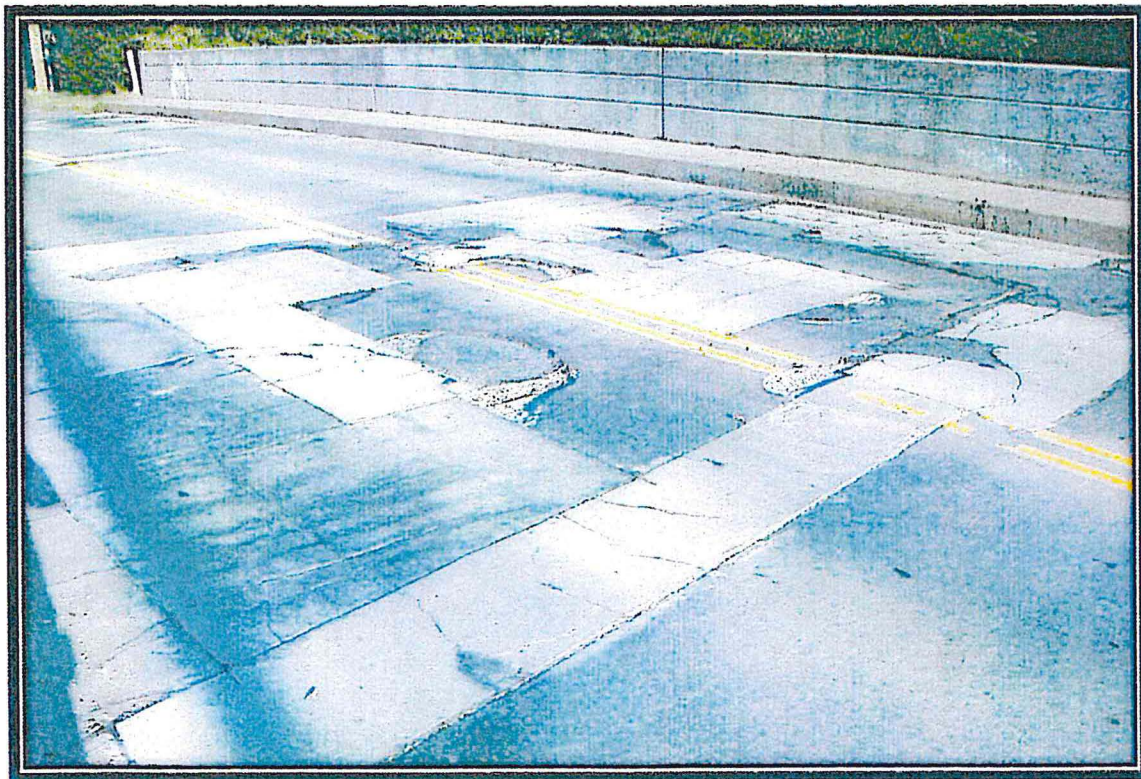
Condition of the Deck
