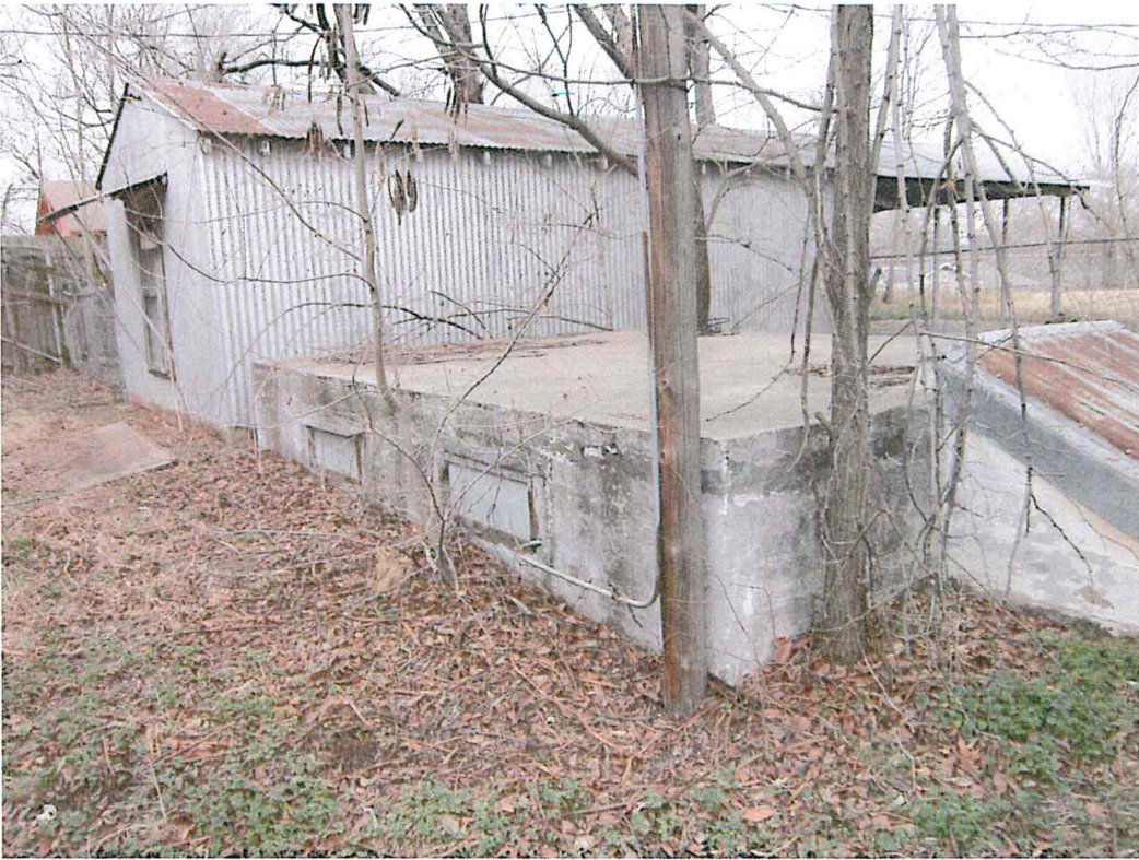
Photo 9: View of carport and storm shelter.
