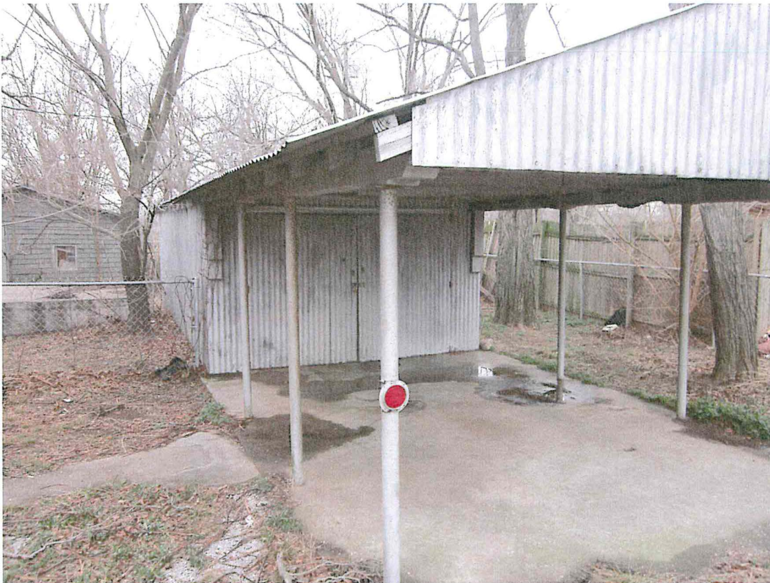
Photo 11: View of carport from front.
