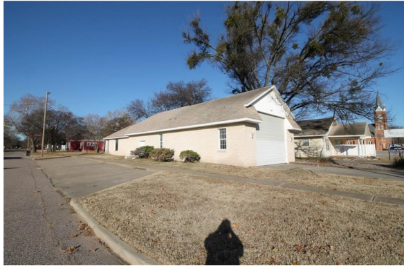
Picture A - Front and side of the Tech Center
