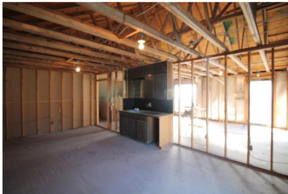
Picture C- Conference room- interior
