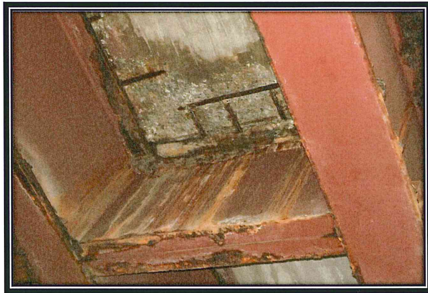
Typical Condition of Soffit at Diaphragms and Fixed Joints
