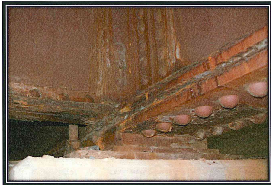
Typical Bearing and Connection Condition
