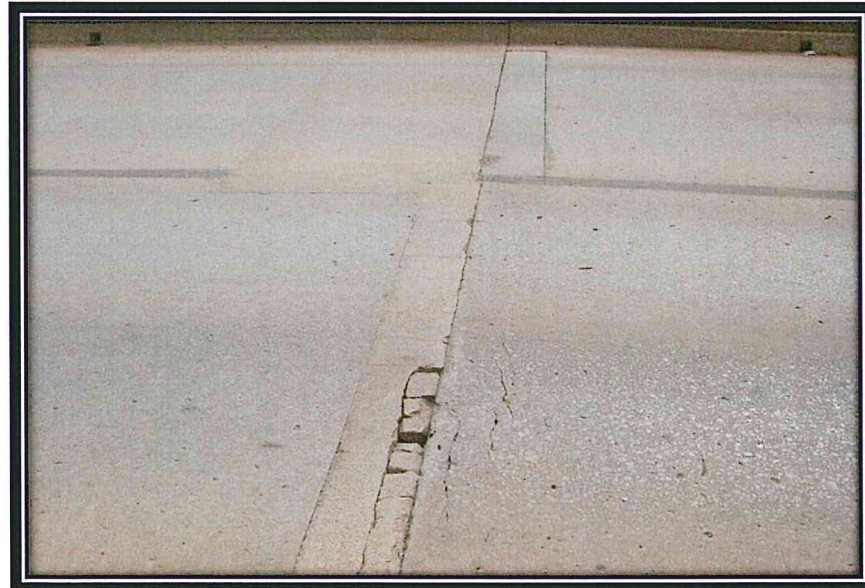
Typical Condition at Fixed Joints and Saw Cuts
