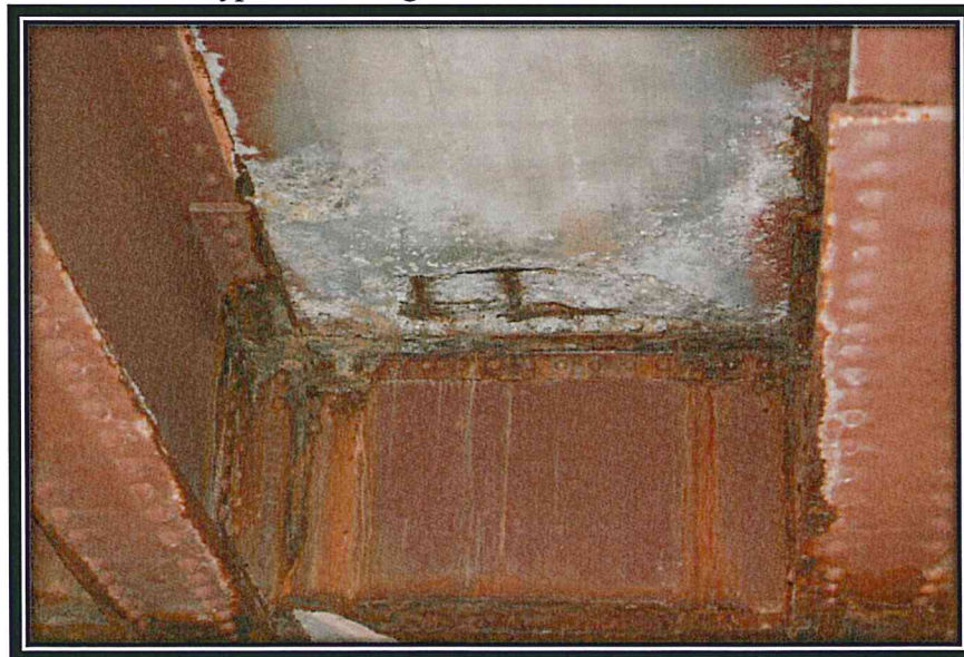
Typical Condition of the Diaphragms and Beams
