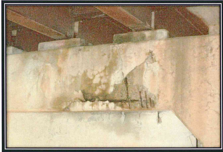
Typical Condition of Pier Caps
