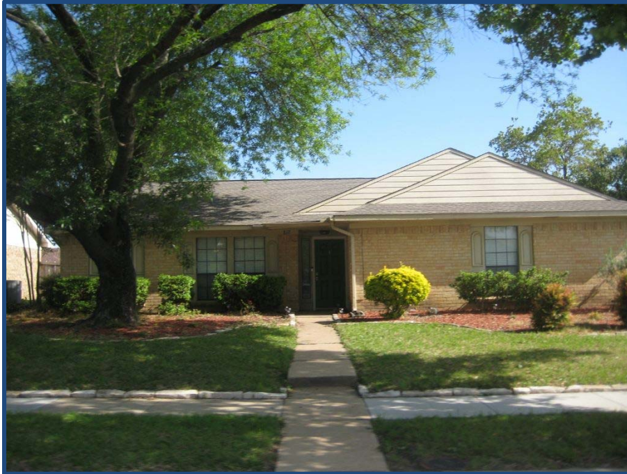
Typical neighborhood home
