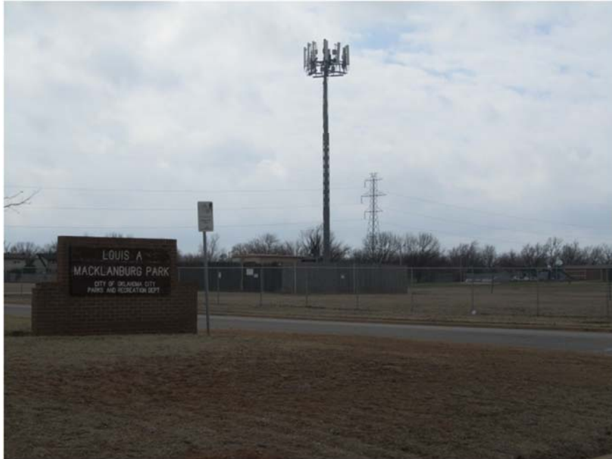
Photo taken from NW 117 th ST, facing toward the monopole
