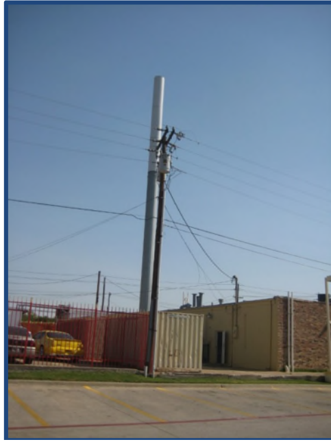
View of cell tower from adjacent Braum's parking lot to its south
