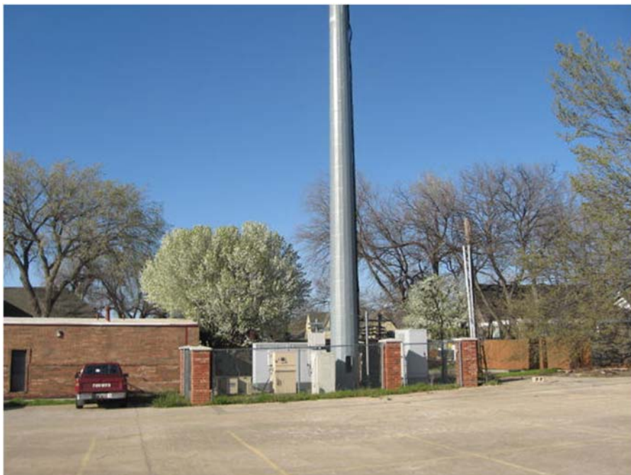
Photo of side view of base of monopole on N Classen Blvd
