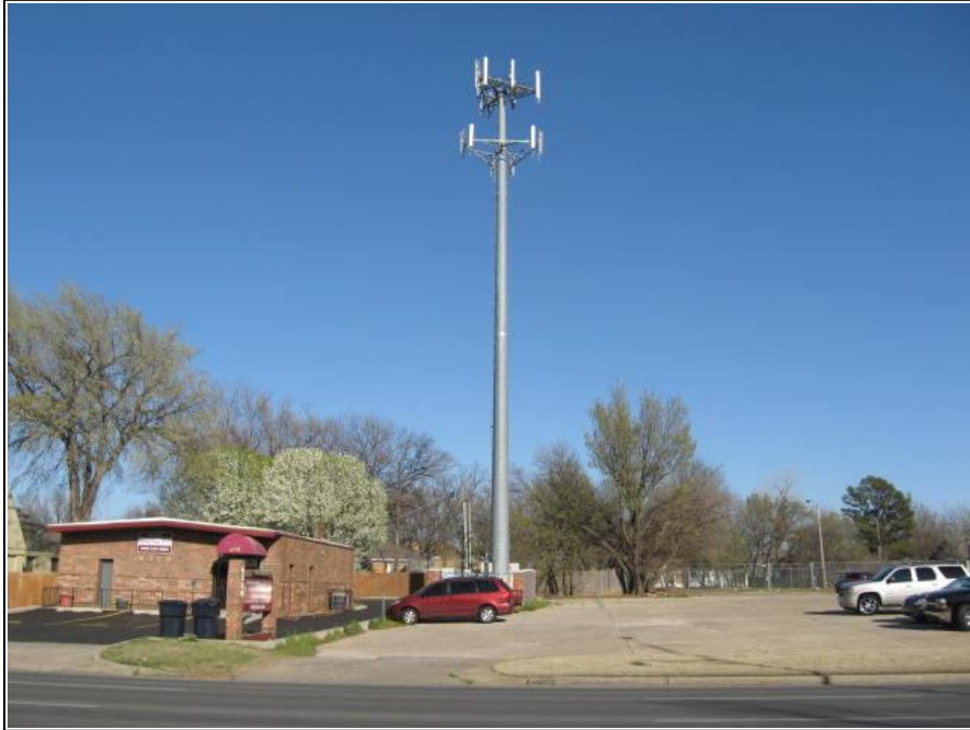
Photo taken of the front of 4312 N Classen Blvd monopole
