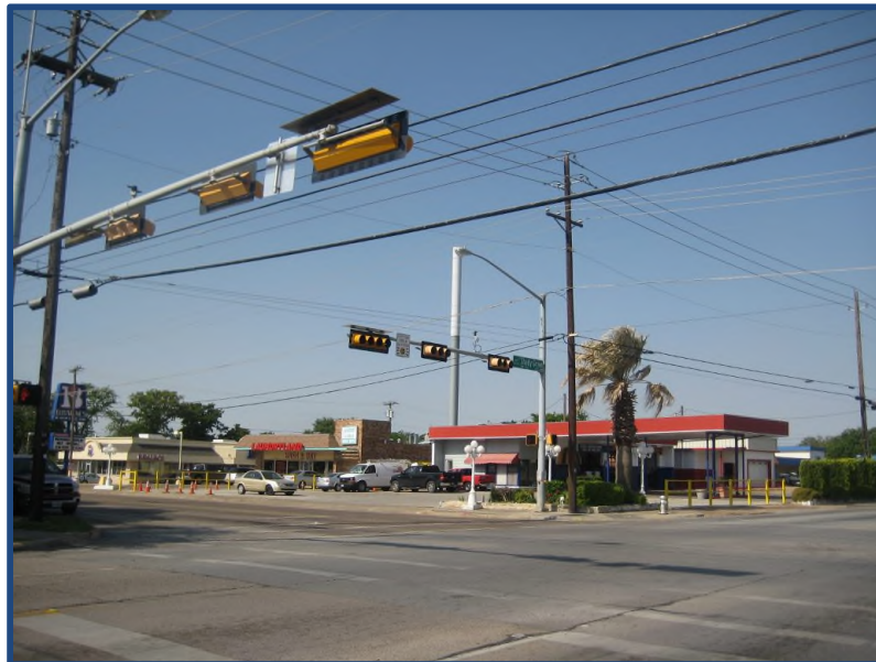
View of cell tower from the NE/C of W. Shady Grove Rd. & S. Story Rd.
