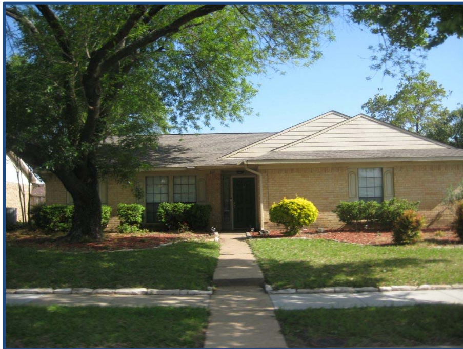
Typical neighborhood home
