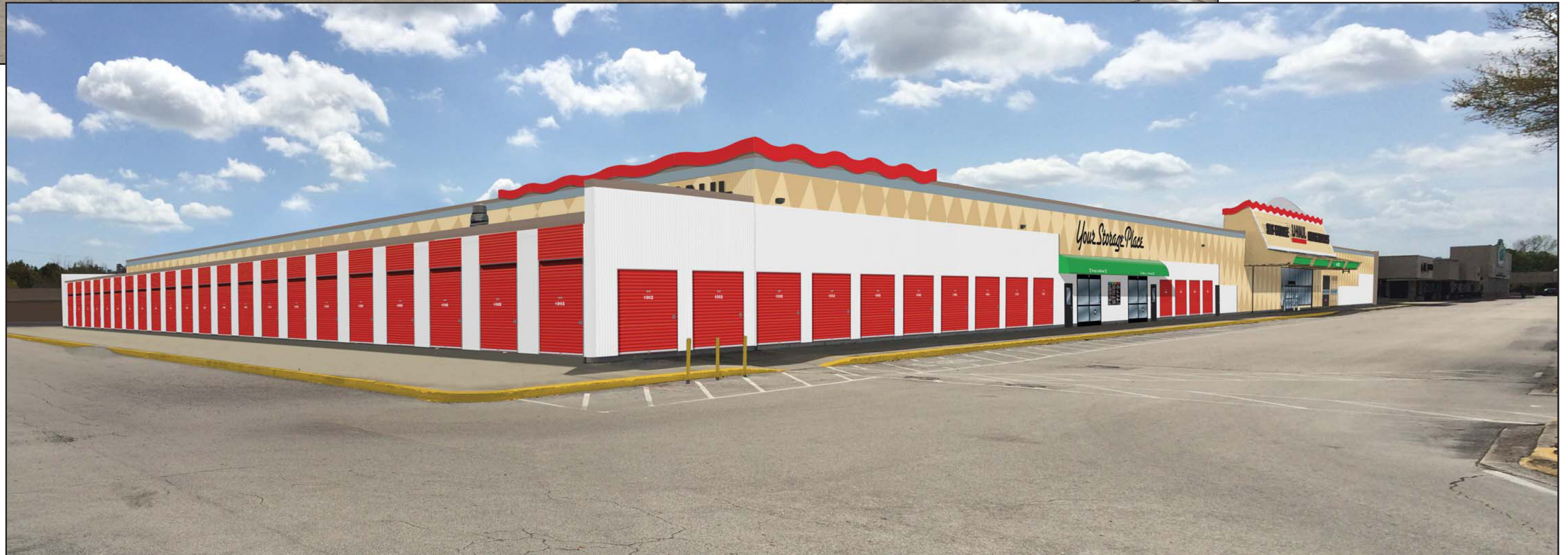
NORTHWEST ELEVATION AFTER
