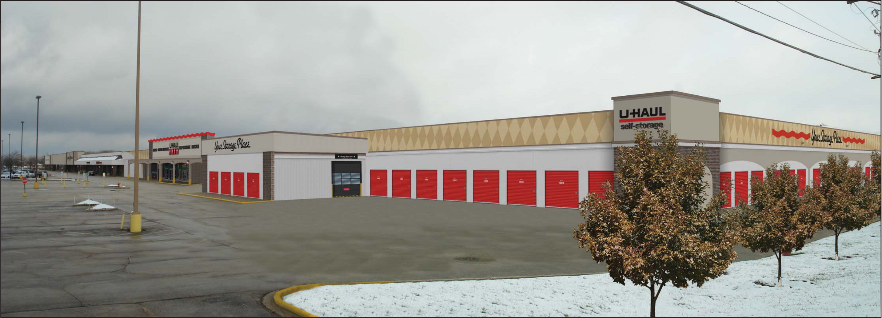
SOOUTHWEST ELEVATION AFTER
