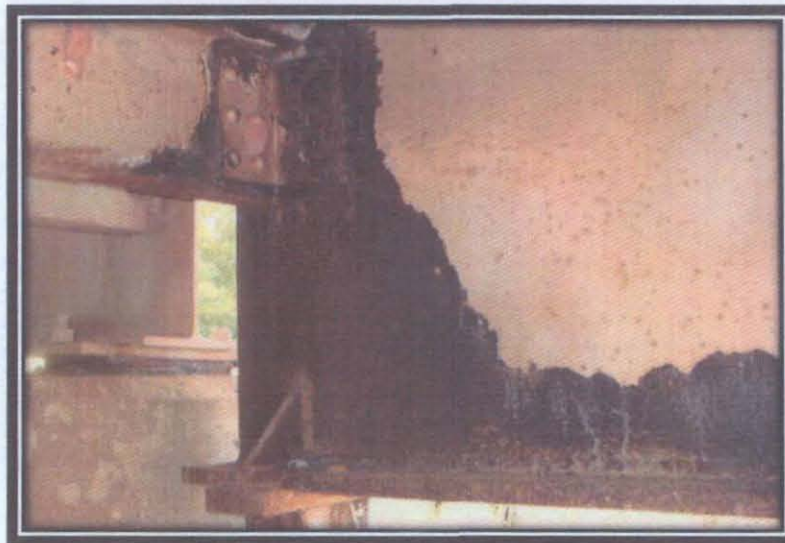
Typical Condition of Beam end and Fascia Beams
