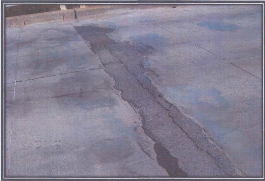
Typical Condition at Expansion and Fixed Joints
