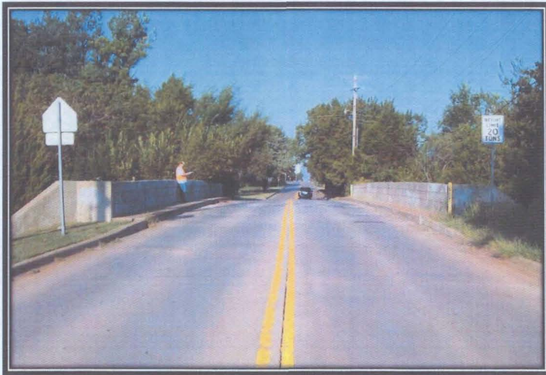
Looking West along the deck.
