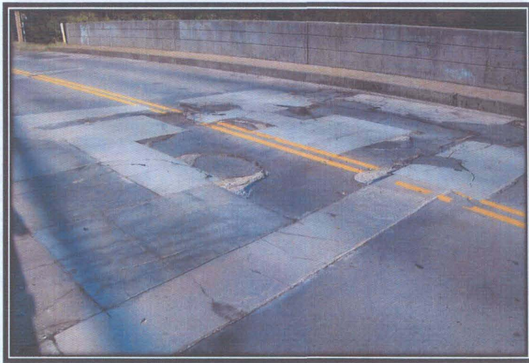
Condition of the Deck
