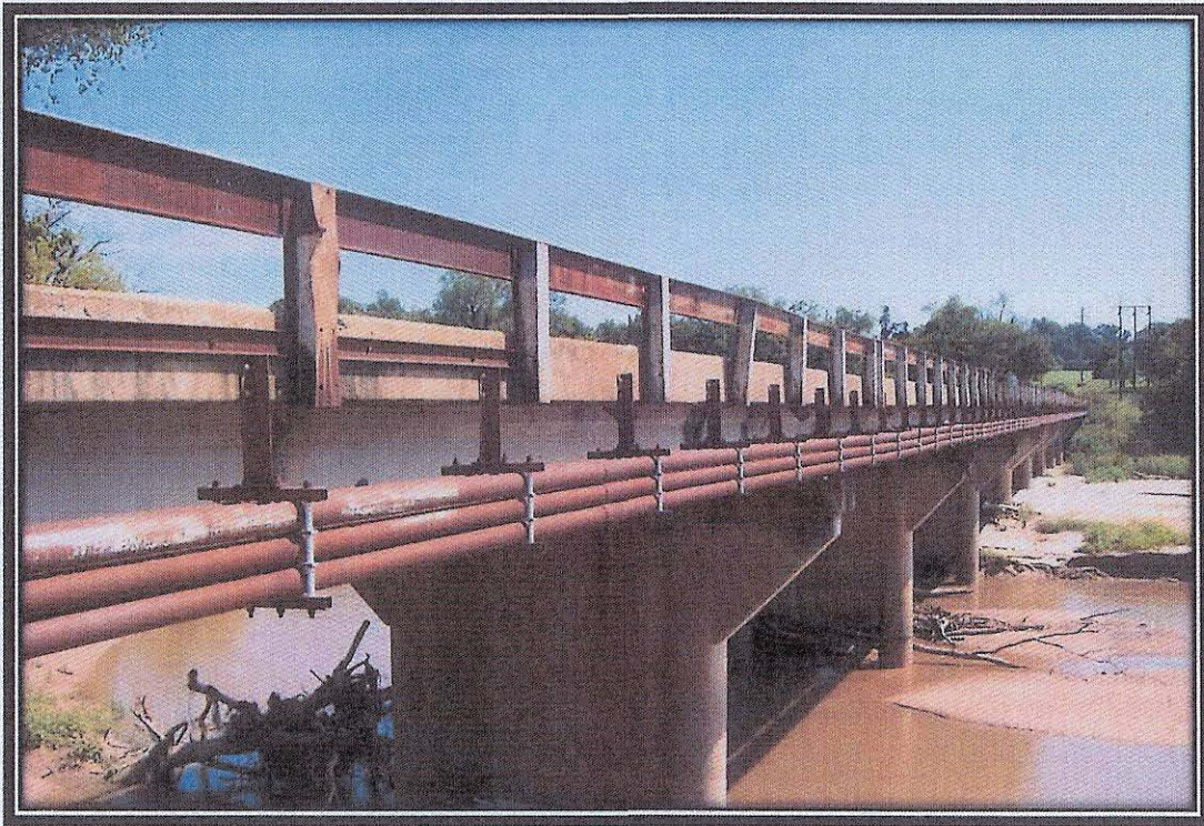
South Profile of Bridge
