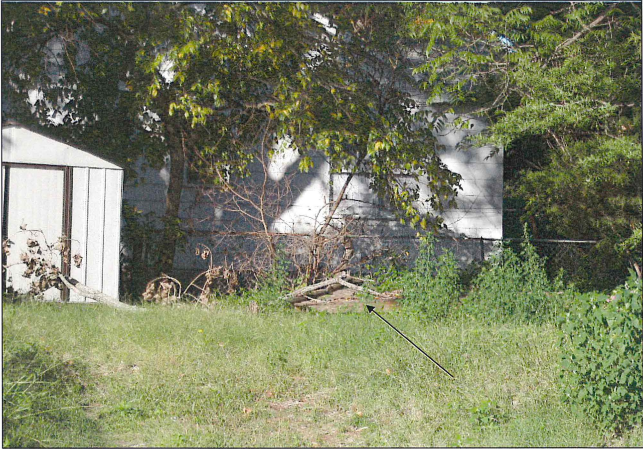
Figure 3: View of wood ramp structure, October 2012.
