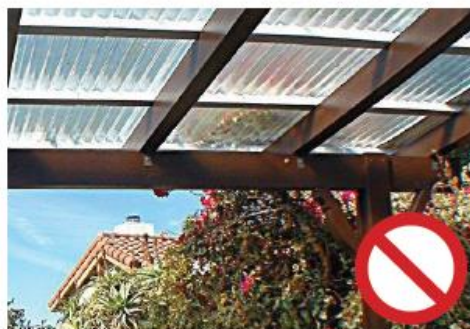
Corrugated plastic is not acceptable
