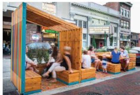
Coated wood planters as barrier walls
