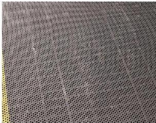
Perforated aluminum floor
