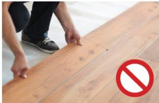
Interior laminate flooring is not acceptable
