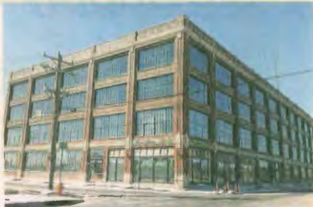
Name of project: 21c Museum Hotel Address: 900 W Main, built in 1916 Total investment: $56.4 million
